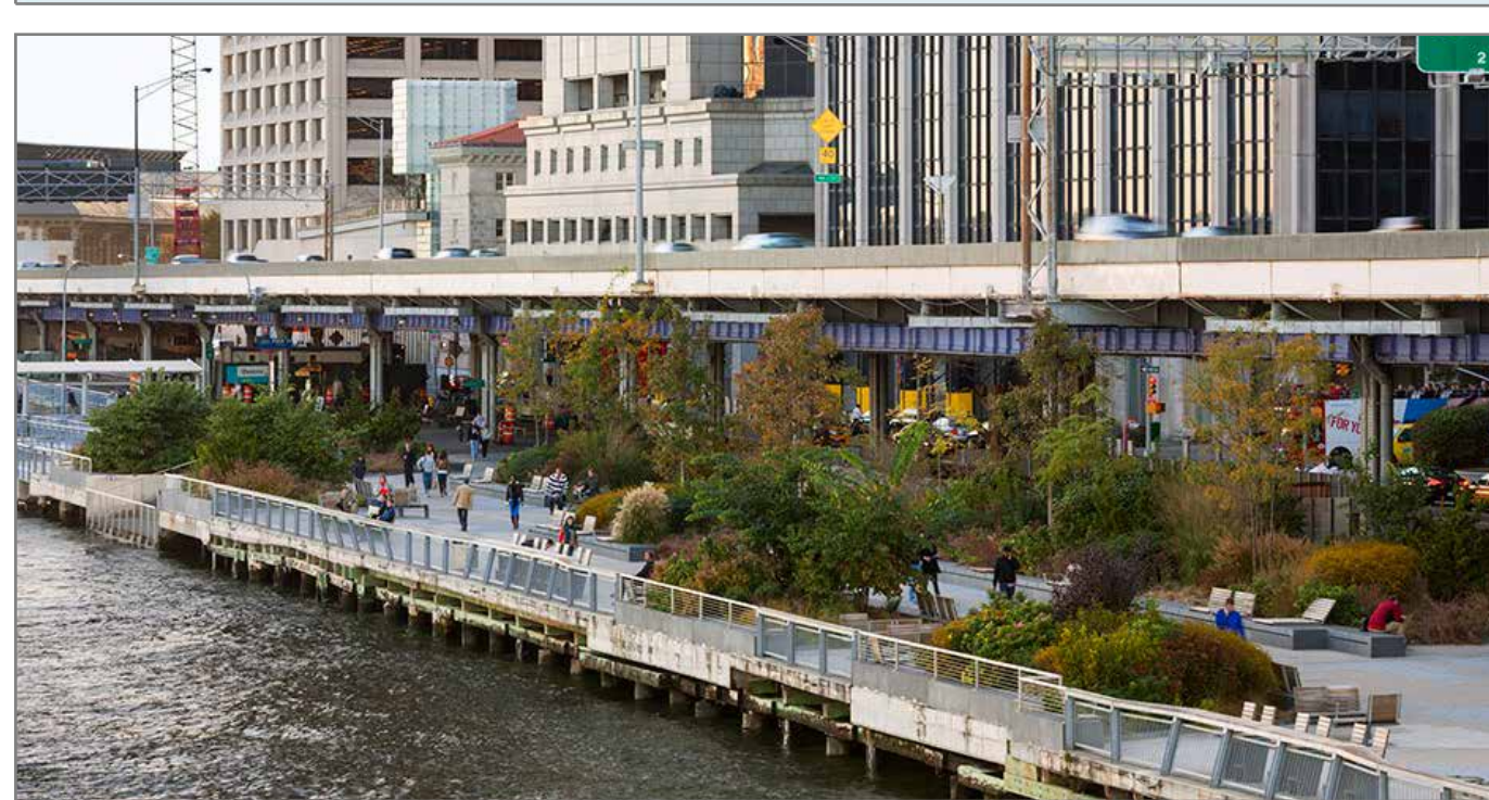
ESPLANADE UNDER HIGHWAY
