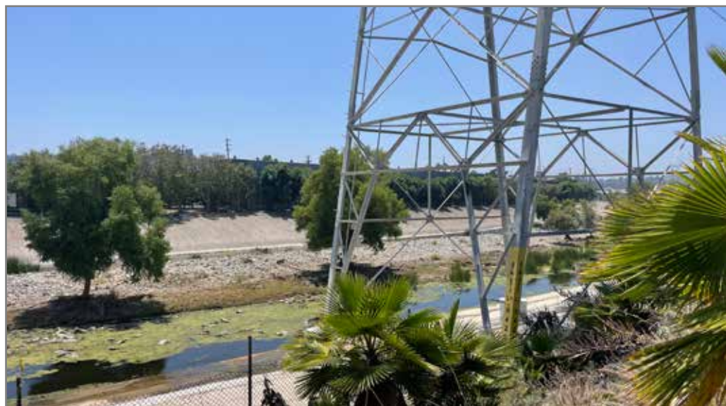
(I) VIEW OBSTRUCTED BY POWER LINE STRUCTURE
