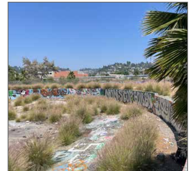
Remaining Turntable Structure
