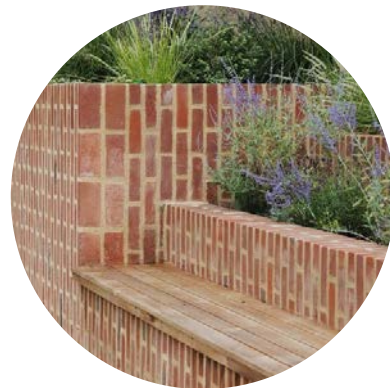
ADDITIONAL BRICK WALLS WITH WOODEN BENCHES DEFINE GATHERING SPACES AND ARE SOFTENED BY NATIVE PLANTS
