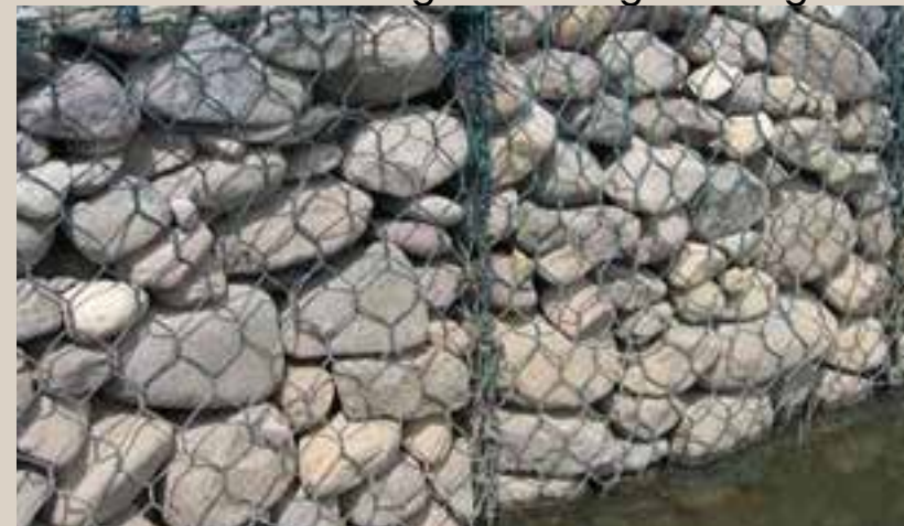
Gabion for retaining walls along river edge
