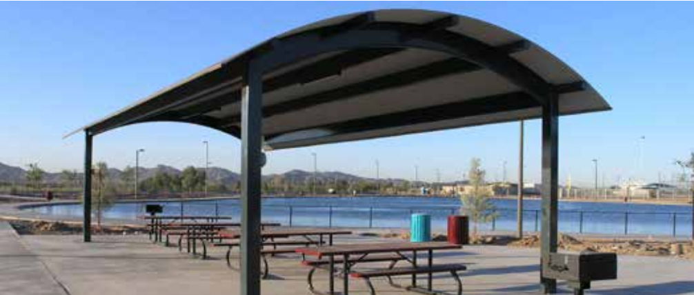
CURVED SHADE STRUCTURE
