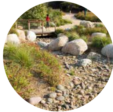
DRY CREEK BED/ BIOSWALE
