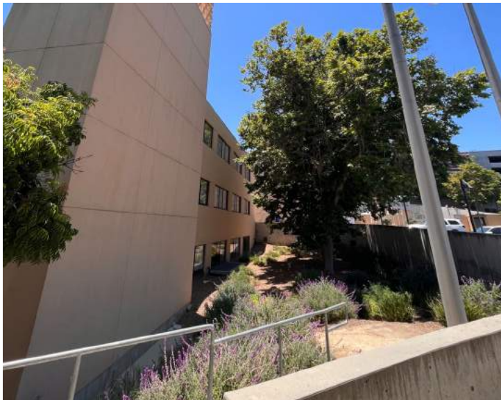
④ Sunken area on west side of City Hall
