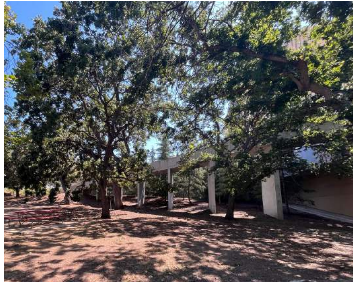
③ View of ramp from below
