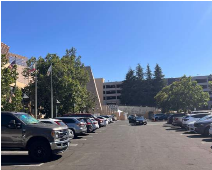
① View from parking lot toward parking structure
