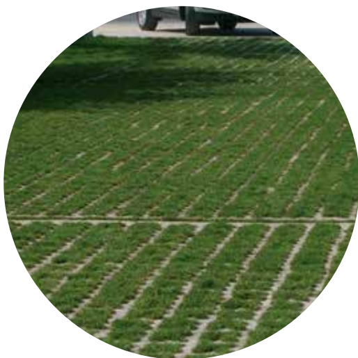
Grass crete suggested use for vehicle loading entrance.
