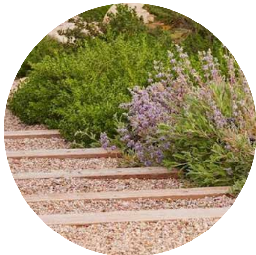
Gravel and wood permeable stairs
