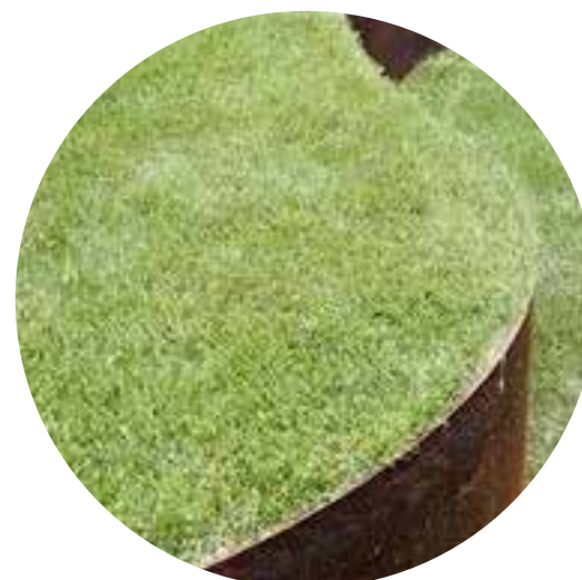
Cor-ten steel used as a retaining wall on Thousand Oaks Blvd and the South side of the park.
