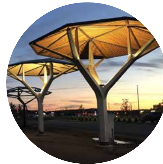
Solar panel light & shade structure
