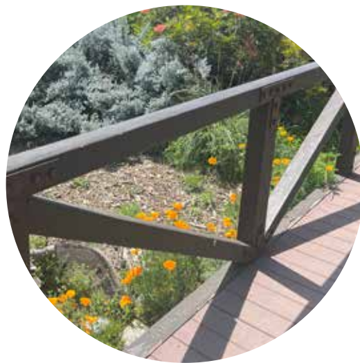
Dry creek bridge
