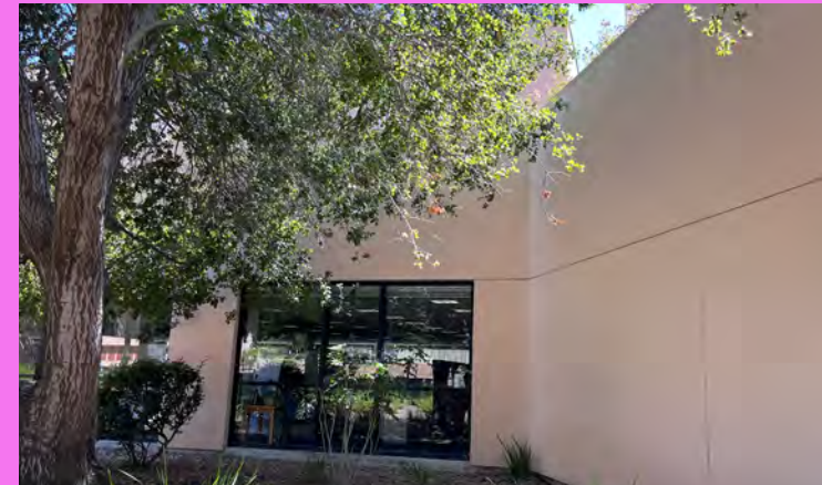
3C Space adjacent to the building is difficult to access and does not provide space for gathering.
