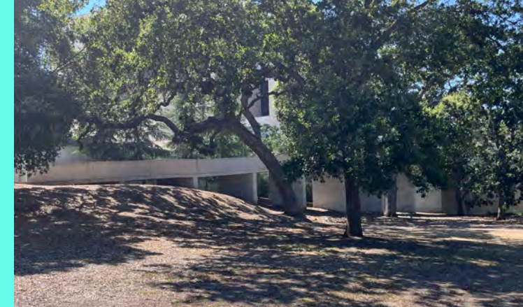
4B The canopy of the protected oak groves presents an opportunity for an outdoor classroom.
