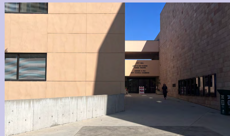
2C The current main entry is difficult to find. There will be a new main entry facing the street.
