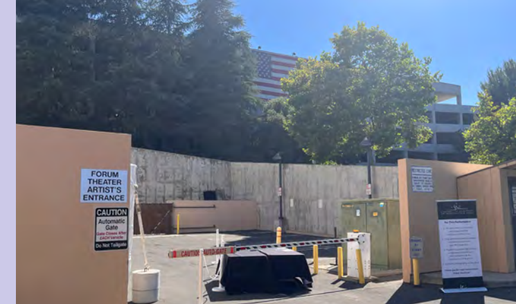
2B The loading zone is unsightly. The entry will be relocated and separated from pedestrian circulation.
