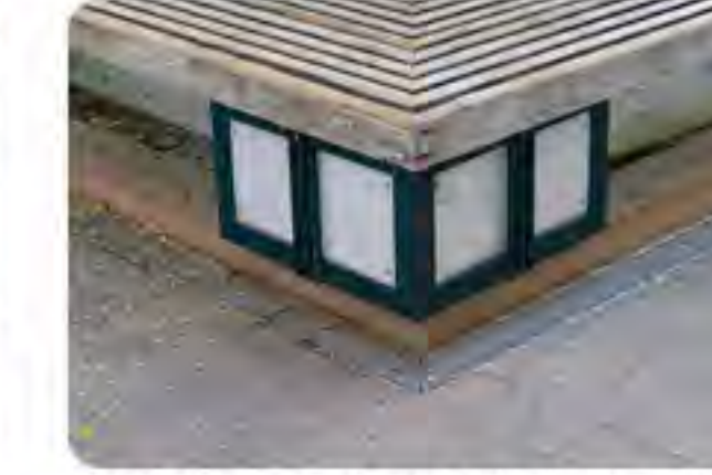
Center bench: Low point with drainage lines around circumference of bench
