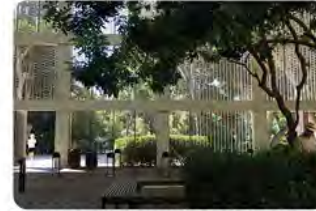
South: View of main entrance from inside the courtyard
