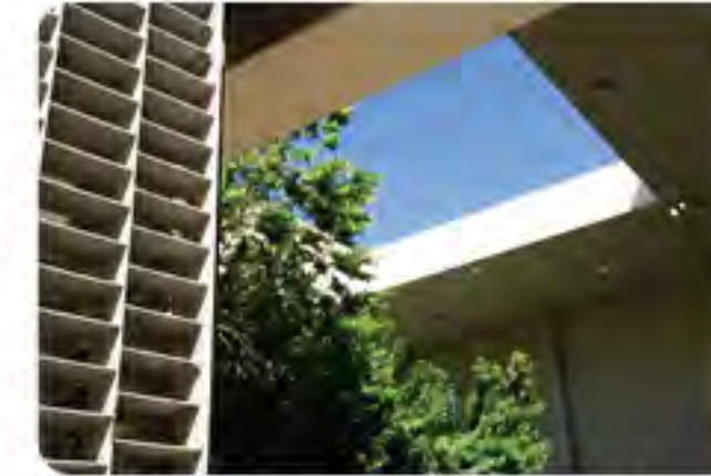
Metal scrim door with view looking up to centered square opening in ceiling
