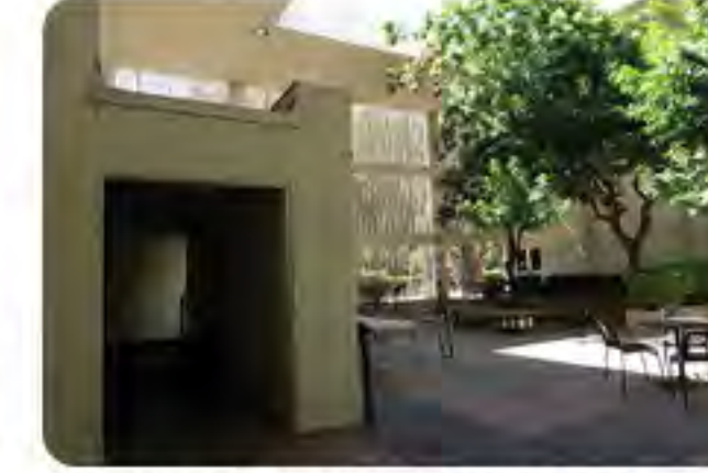
Singular use of vestibule to block noise and light from theater, with ramp and stairs up.
