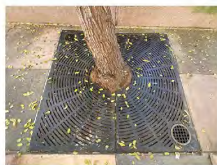
Tree growth is being constricted by paving, compacted soil, + drainage grates
