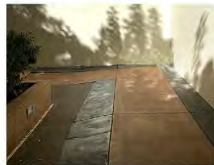
Inverted slope leads rainwater to drainage point at center of the site
