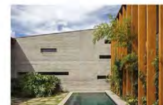
Update brise soleil to allow for planting along south side of space
