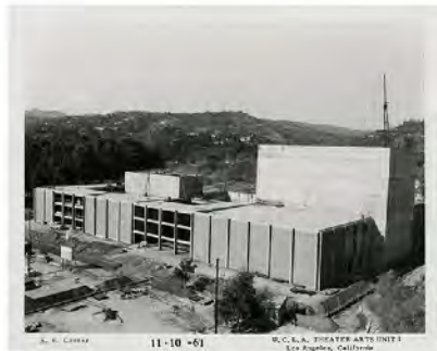
Construction of Macgowan Hall: November 1961
