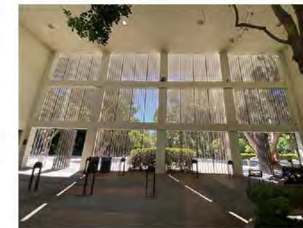
30' tall courtyard walls and metal scrim restrict views out to Murphy Sculpture Garden
