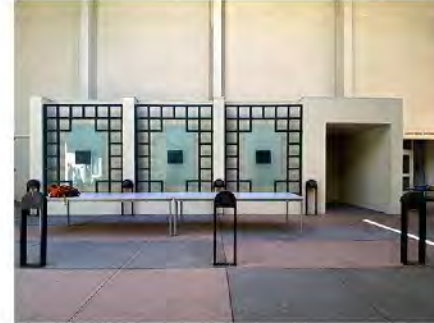
Vestibule is uninviting + breaks up site symmetry Purpose is to keep light + sound from entering Freud Playhouse, but is a visually distracting area when not in use
