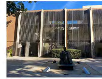
View of courtyard entrance from Murphy Sculpture Garden. Brise soleil wall is a key feature in the current design + serves as the main pedestrian access to the space
