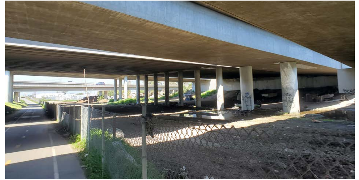
D: 91 Freeway underpass and bike path
