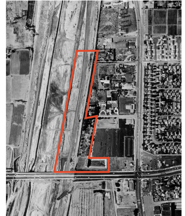
1956: LA River channel under construction
