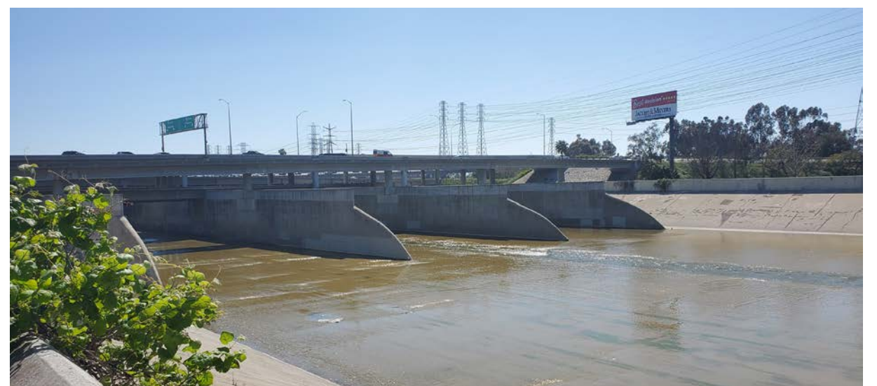
F: Artesia Blvd bridge at LA River
