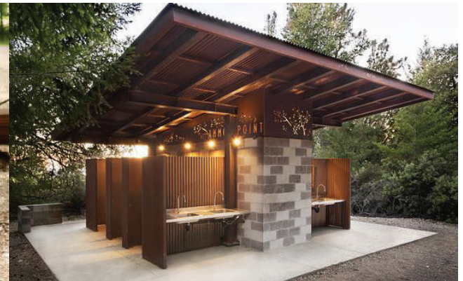
Beautiful restrooms and wash stations.
