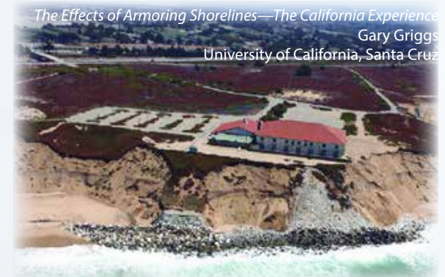
The Effects of Armoring Shorelines—The California Experience Gary Griggs University of California, Santa Cruz Stilwell Hall at Fort Ord, built in 1940- removed in 2003 due to coastal erosion
