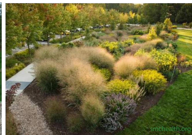
Infiltration bioswale (0.3 ac)
