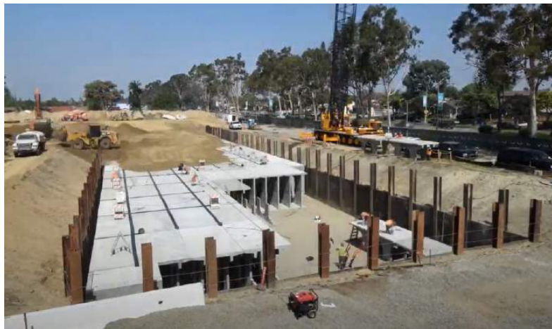
The underground stormwater collection reservoir (2 ac)
