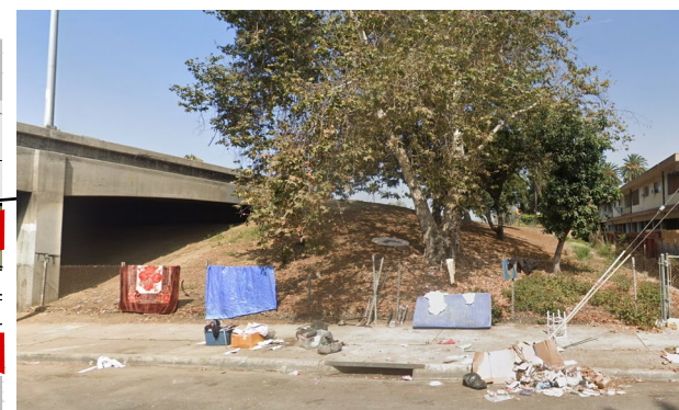
Freeway embankment @ Coronado St.
