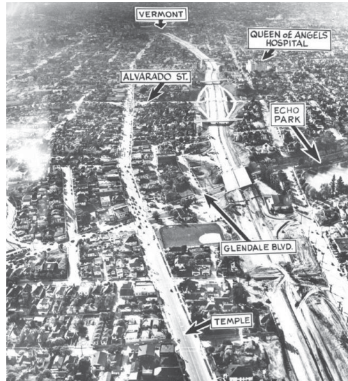
Aerial view looking west towards Hollywood shows the partially completed Hollywood Freeway. New freeway runs parallel to Temple, then converges near Vermont. April, 1950.
