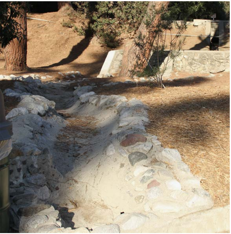
PROPOSED REDESIGN OF DRAIN SYSTEM First, complete excavation. The concept is to make this area more natural, and more sustainable. Re-grade to make 4 Berms (2 on each side) that flow into a new central down sloping Bioswale that is lined with river rock and follows the style of the CCC-man-made boulders throughout the Dell. Plantings of shrubs and California natives would provide habitat and nutrients to the soil, encouraging improved soil composition and facilitate the decomposing of a more diverse plant material. A main drain at the parking lot edge would push the water below the surface to underground cisterns located in the parking lot under the permeable pavers.
