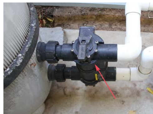
Flow detector valve
