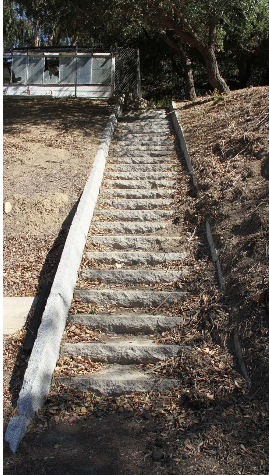
The steps to no where. Hand carved granite steps, built sometime in the 1930s, used to lead to the upper greenhouses at the east side, top of the slope. Obviously not to today's code, with no handrails.
