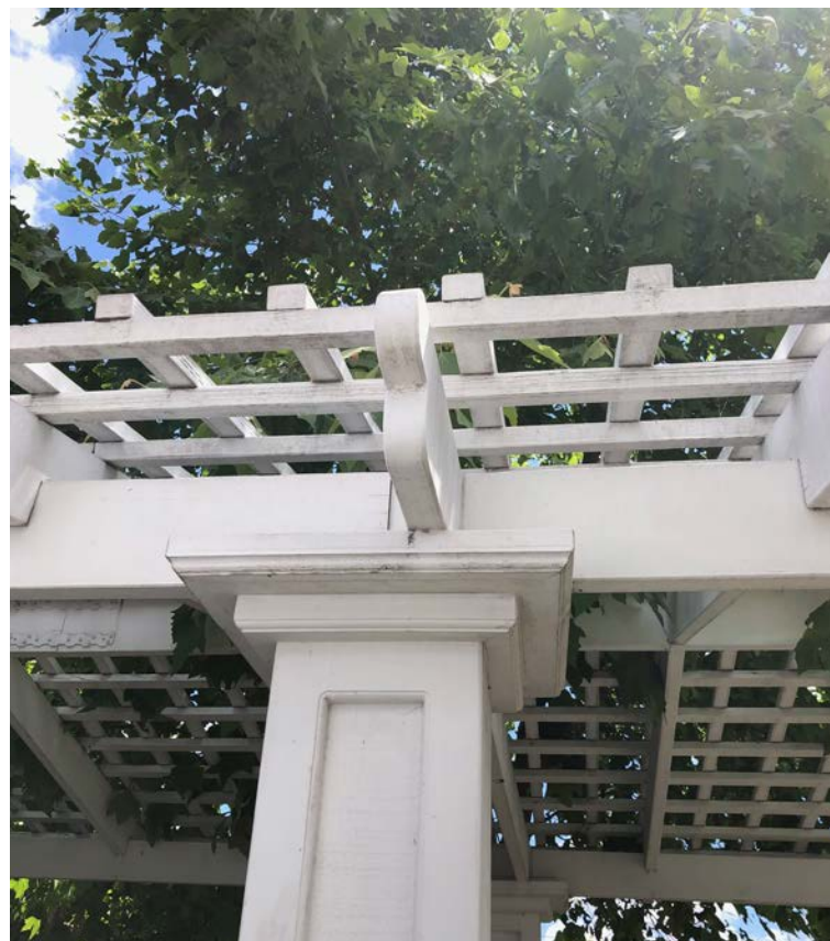
Side column detail
