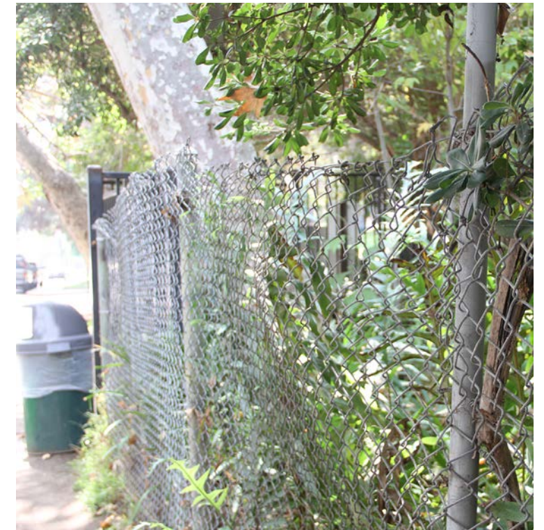
Ineffective and unattractive fencing
