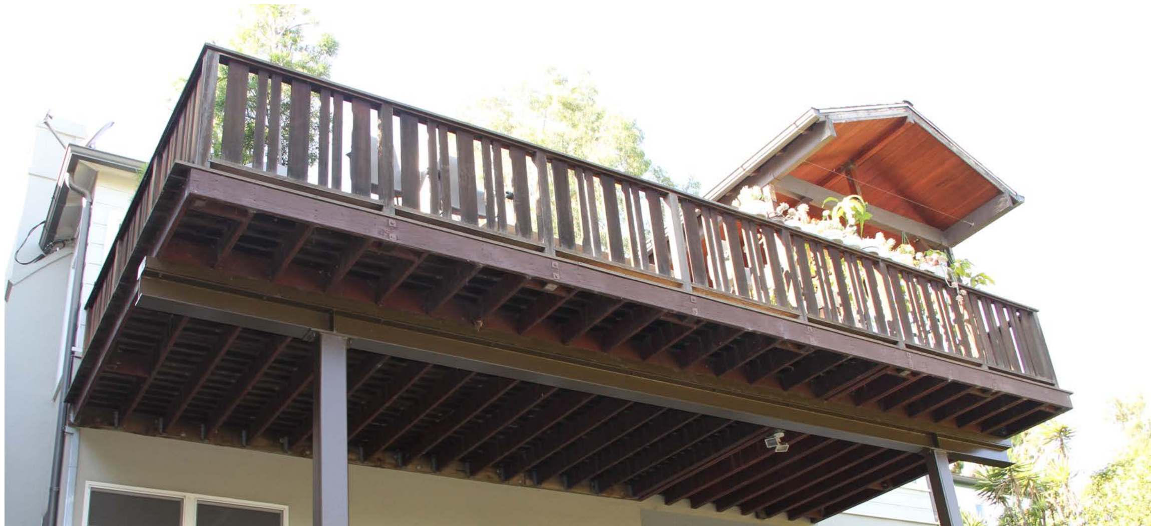
The deck (approx. 31' x 17' includes a shade cover and railings).
