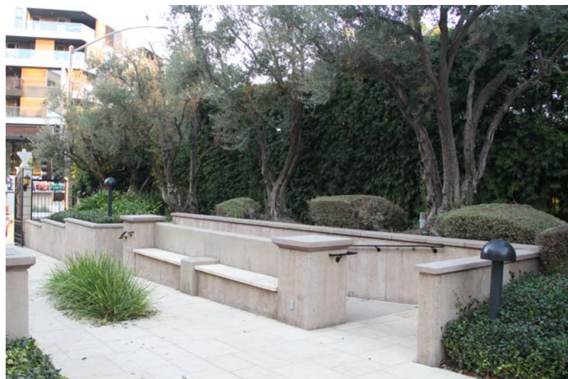
Planter wall at gate entrance, with ramp and bench
