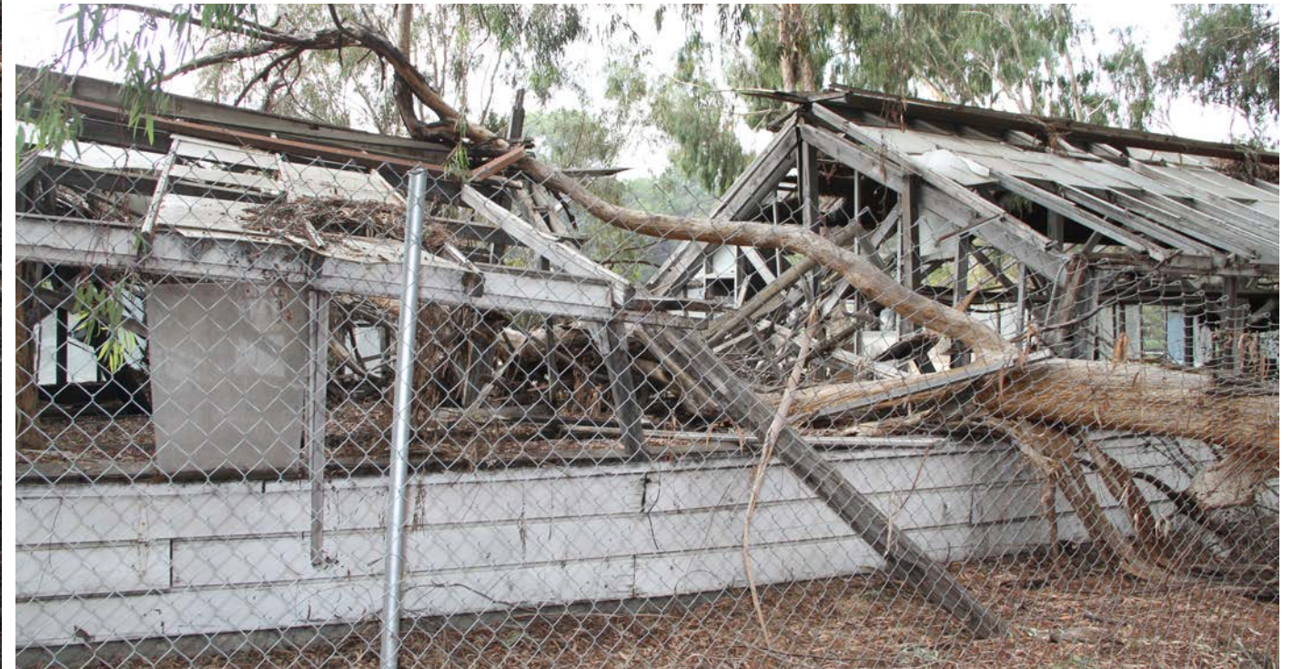
An example of one of the abandoned greenhouses.
