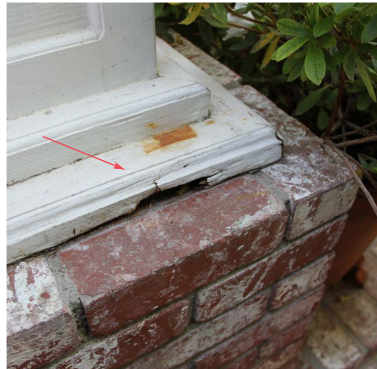
Base of column: Dry rot, water damage
