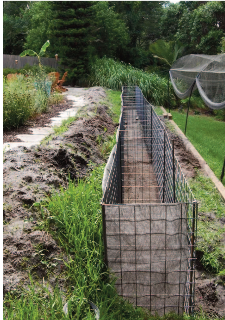
Gabion baskets with geotextile attached, ready for stone placement.
