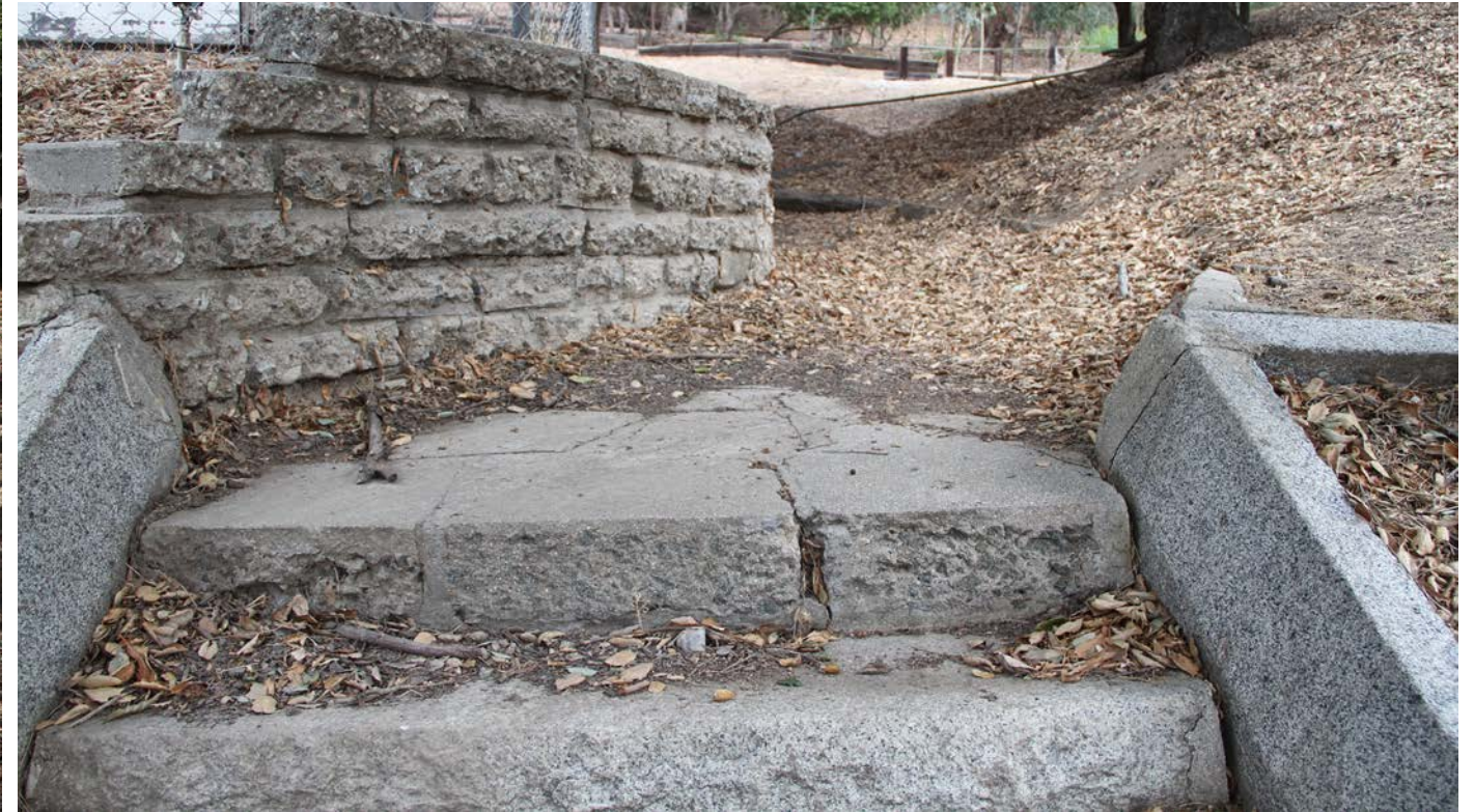
Cracked and crumbling at the top.
