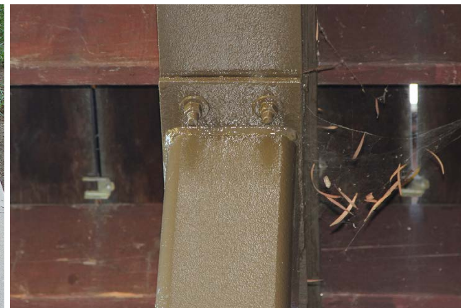
I-beam and vertical beam connection, bolted
