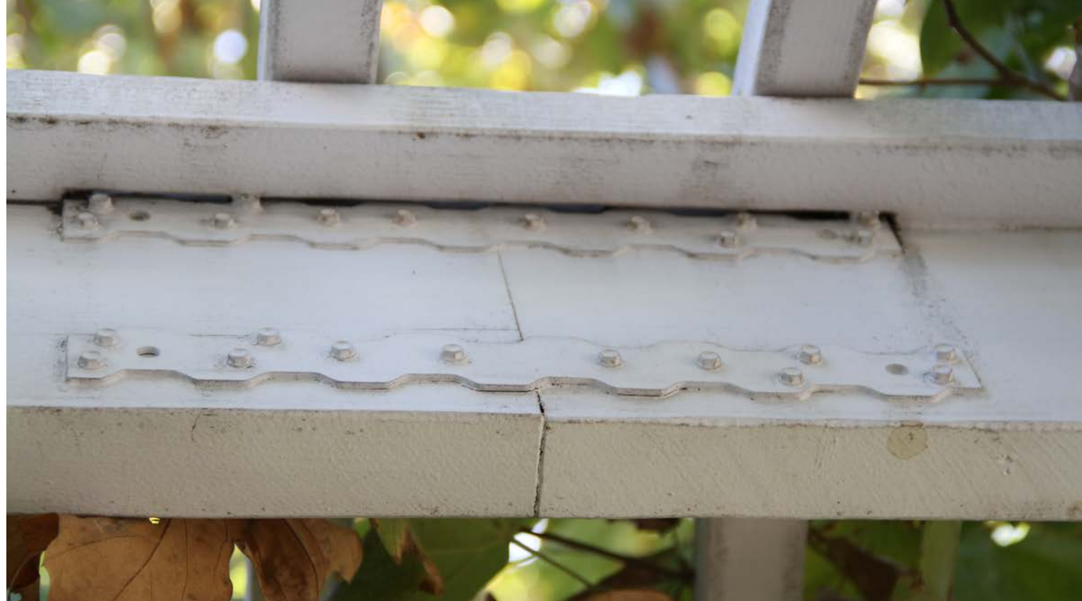
Main support beam extension: 12" Zig Zag Plate Tie. On both sides, least obtrusive hardware selection to join the beams.
