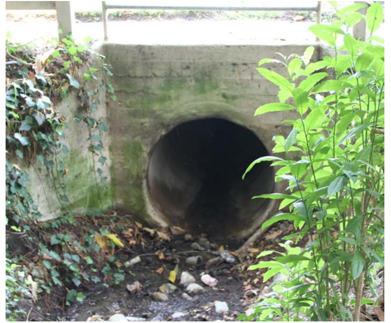
Lower Dell Existing storm drain at Los Feliz Blvd. Channel needs sediment clean-out. Cement is cracked and decomposing.
