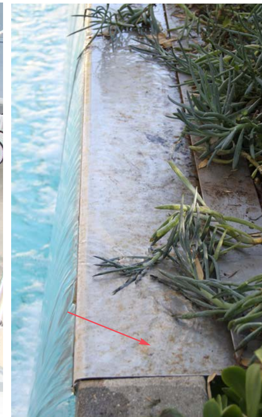
Stainless steel showing saltwater pitting
