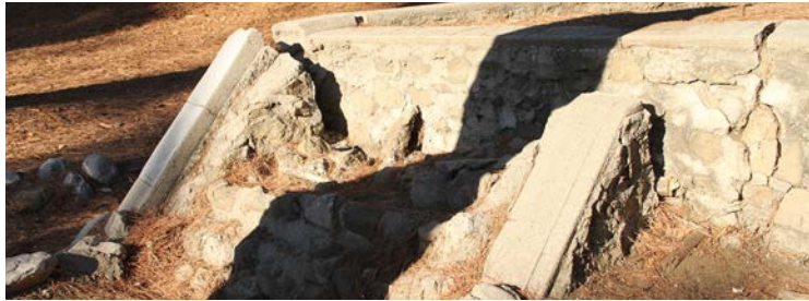
CURRENT STATE OF EXISTING DRAIN SYSTEM Located at the top of the highest parking area in the Upper Dell, this drain system is inadequate at best. The catch basins are full of soil and plant debris, the walls are crumbling and insecure. If it does drain, it flows into the parking lot to the east, which then flows into the man-made catch basins that mimic a creek bed above the playground.
