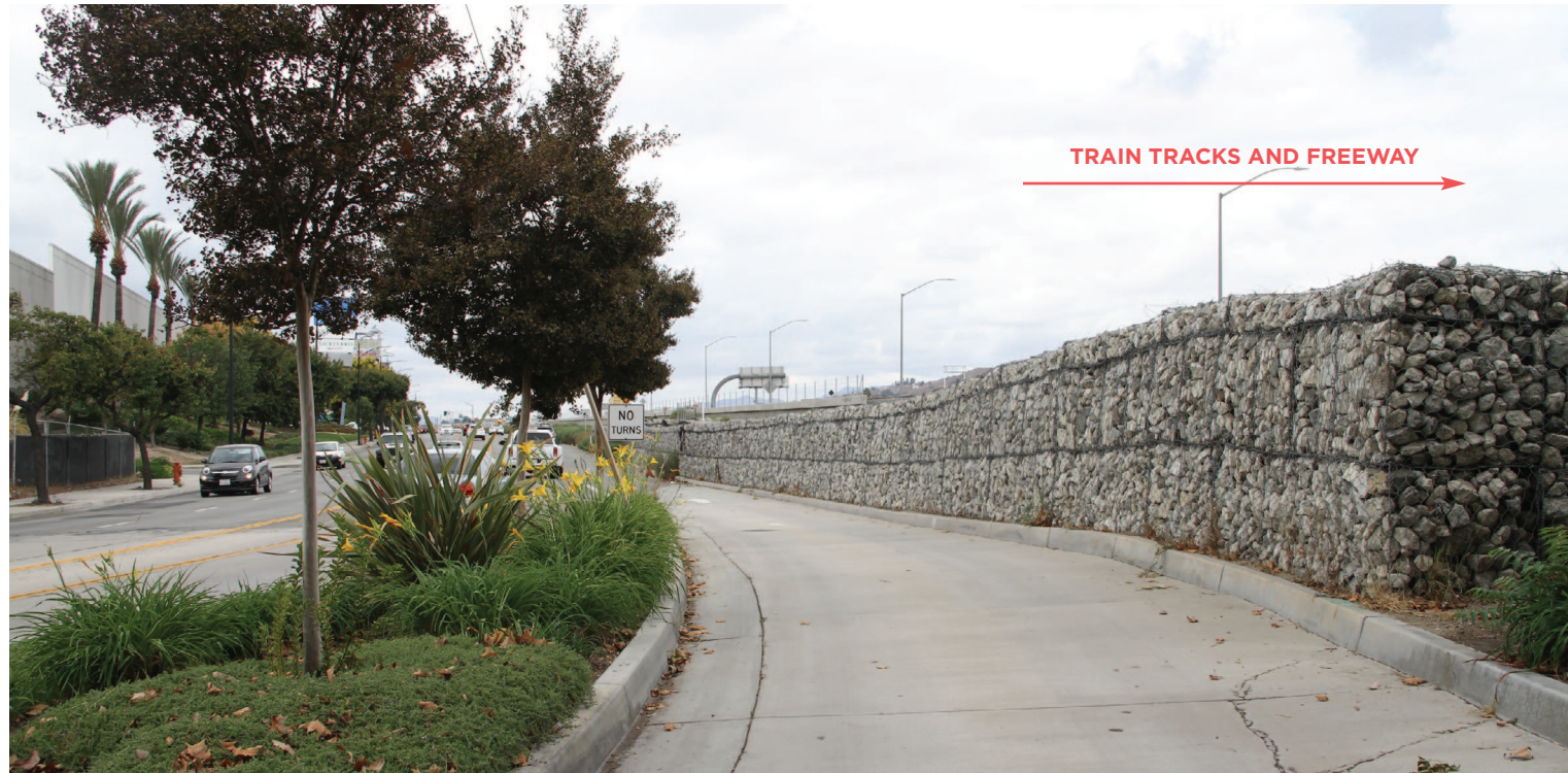
The Gabion retaining wall borders an outlet/merging road from the Animal Shelter onto Victory Blvd. It is supporting the bank of earth that juts up to the train tracks and the I-5 freeway to the east, about 8-9/10 of a mile away.
