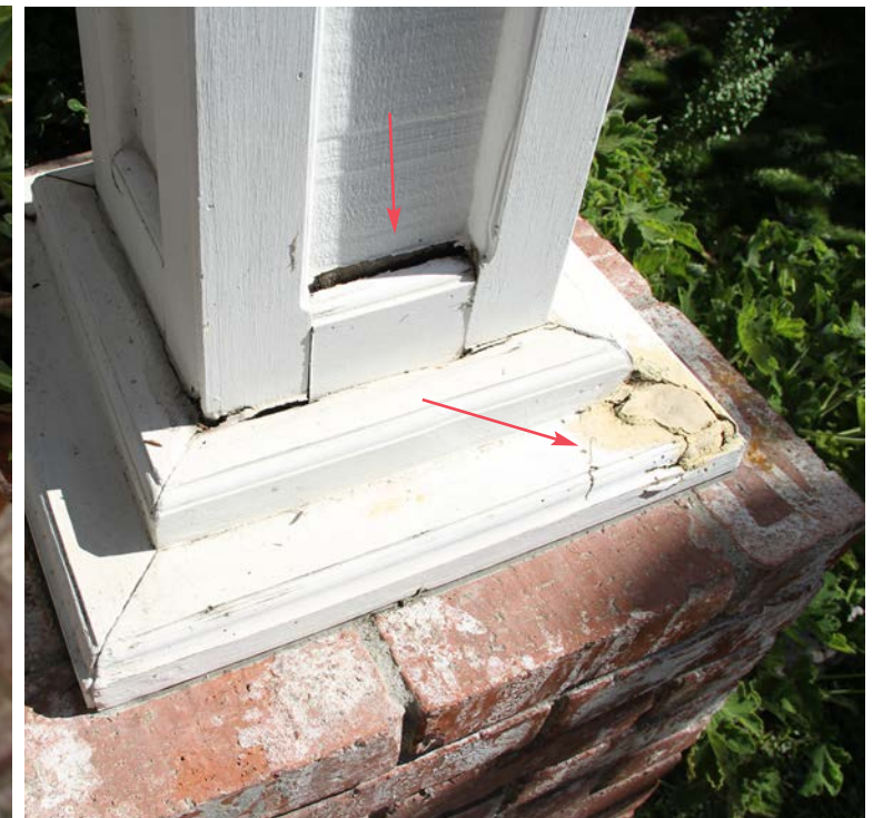
Base of column: extreme water damage
