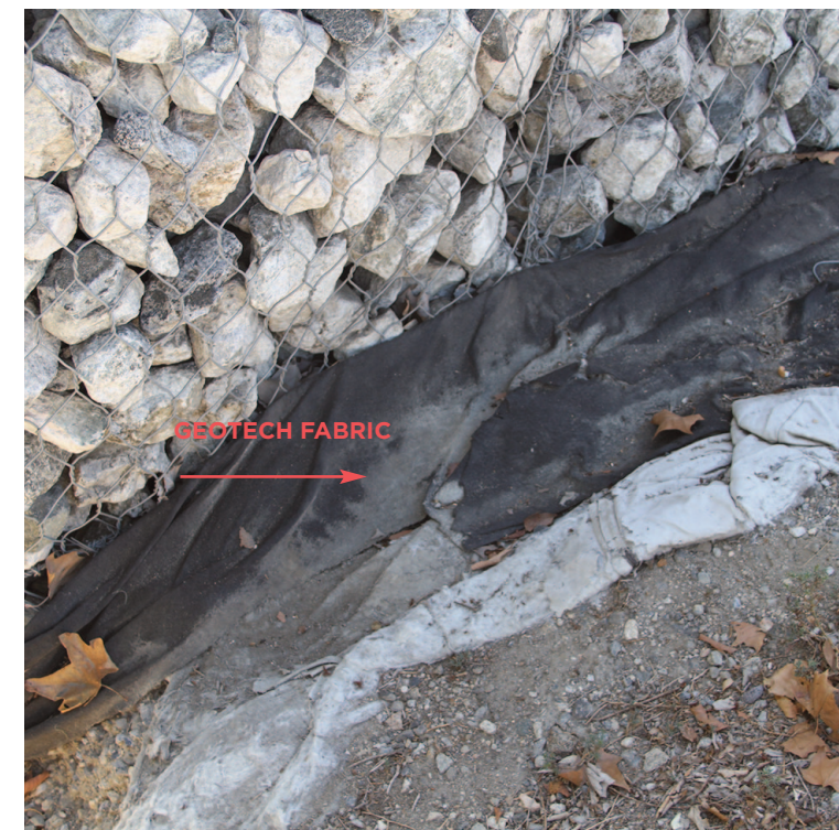
Detail of geotextile filter fabric at the base. Geotextile filter fabric stops fine silts and clay migrating into the wall. The filter fabric ensures the gabion remains free draining, and eliminates hydro-static pressure behind the retaining wall.
