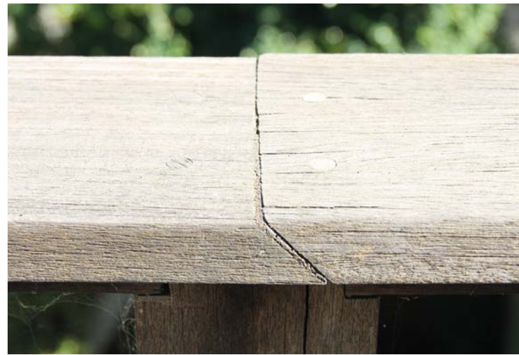
Toe-nailed top of handrail
