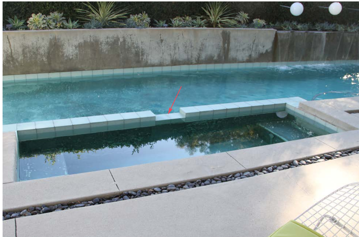
Spa showing edge with overflow notch in tile edging
