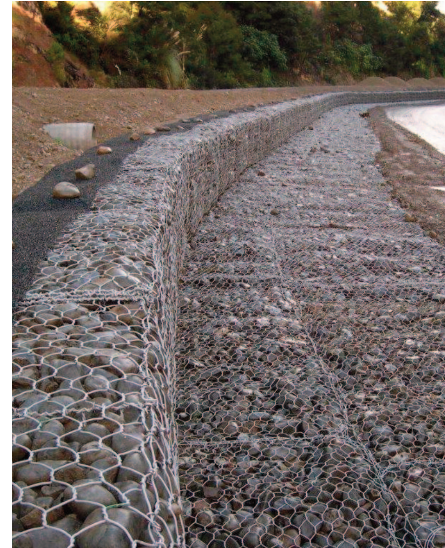
Gabion at top, and mattresses lining the waterway, at the waterway edge.
