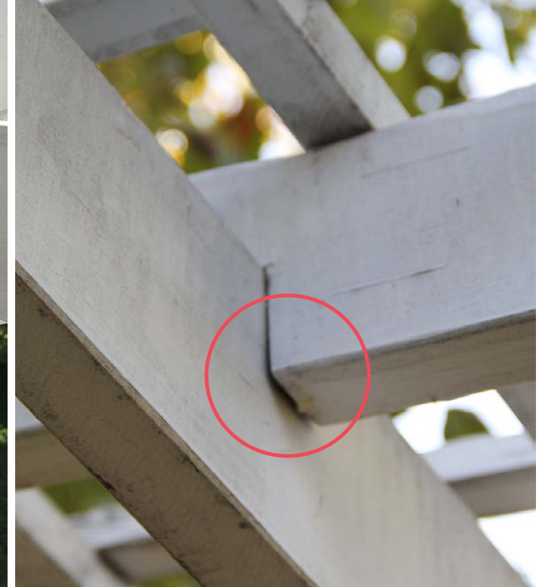
Joist to rafter: Toenailed notch has warped
