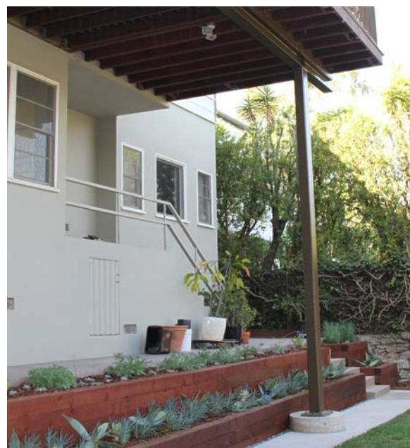
Full view of vertical 15' beam support
