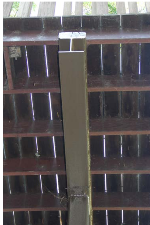
Painted iron I-beam with 4x10 treated Douglas Fir support beam on top.
