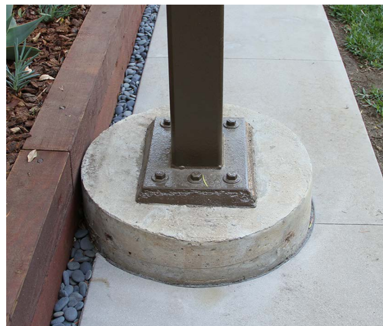
Vertical beam support in concrete column, centered in metal post connector, bolted and epoxy-glued onto concrete
