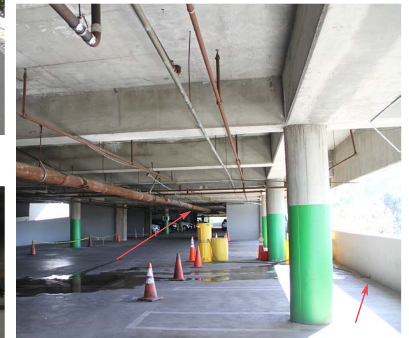
Drainage pipe system under the planter boxes, showing leaking pipes, capture system and drain through weep hole to the slope below.
