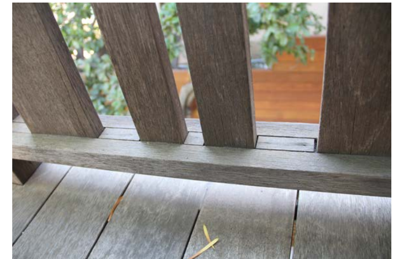
Blocking at base rail where balusters attach
