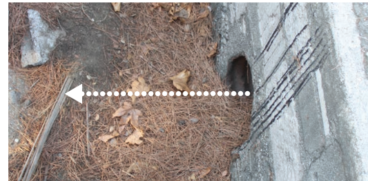
Concrete pipe from under the street going into the catch basin. Basin is full of sediment and rocks.
