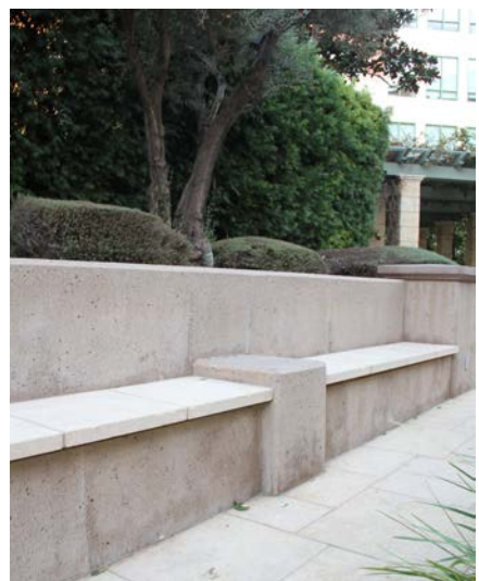
Planter wall with benches
