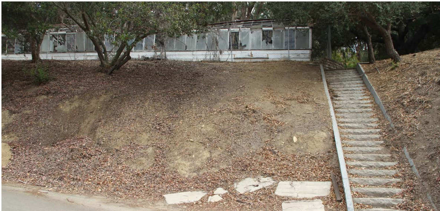
Site where improvement is needed. Greenhouse at top, steps at the right. Olive and oak trees hanging on in the eroding slope area.
