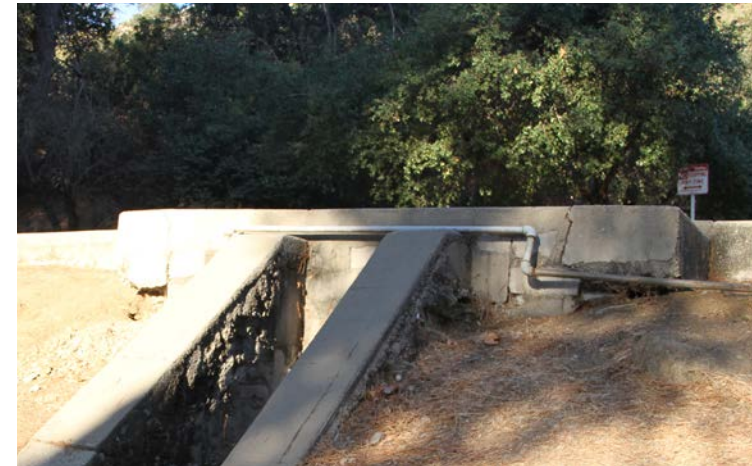
Upper Dell Existing catch basin at top of slope. (upper Dell) Cement is cracked with sprinkler pipes are wrapped around it, some non-functional.
