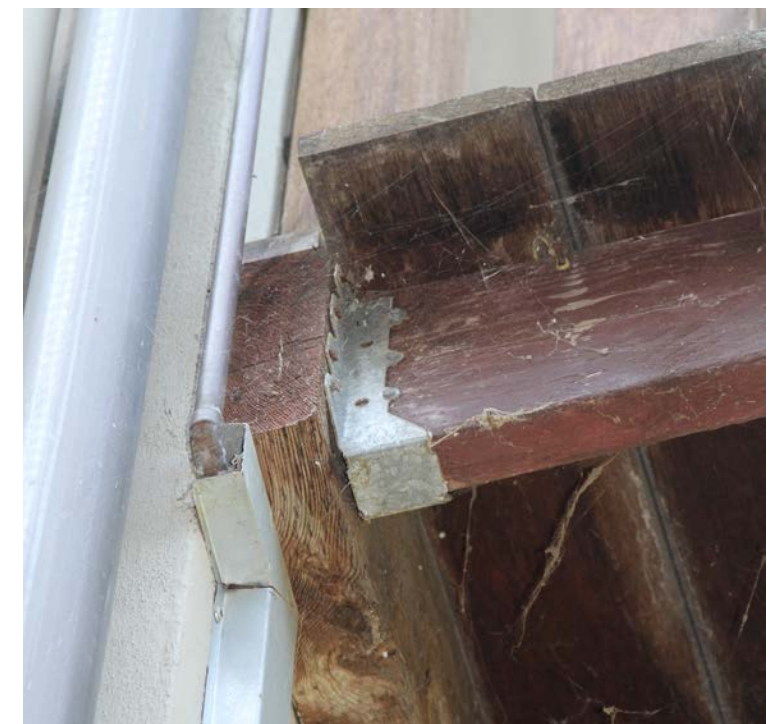
Galvanized steel joist hangers attached to ledger board
