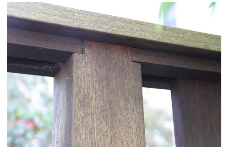
Railing at top of slotted post
