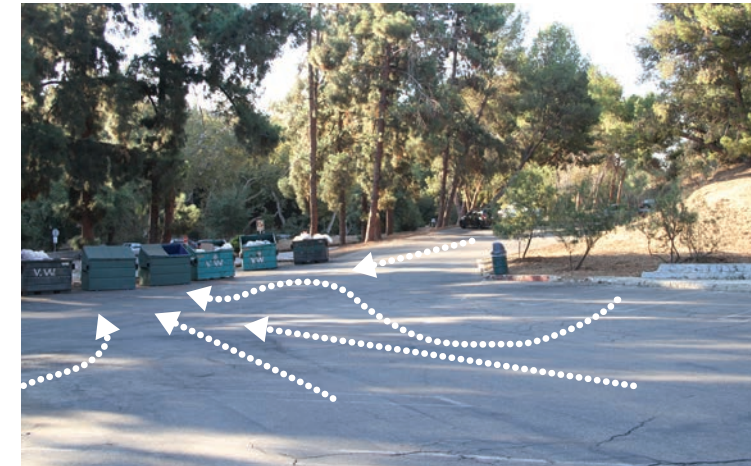
Wide area of parking lot that is cracked and full of hazardous crevices. Should be replaced with permeable paving when pipes are put in for transfer of water from slope to cistern. Water flows into dumpsters.
