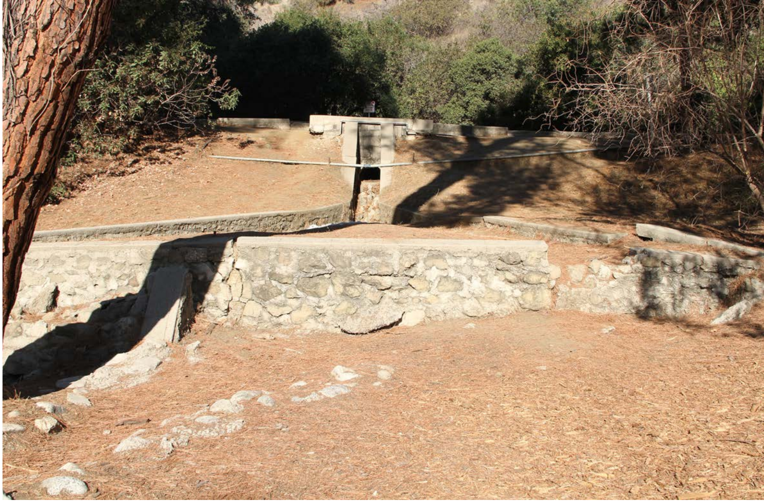
CURRENT STATE OF EXISTING DRAIN SYSTEM Located at the top of the highest parking area in the Upper Dell, this drain system is inadequate at best. The catch basins are full of soil and plant debris, the walls are crumbling and insecure. If it does drain, it flows into the parking lot to the east, which then flows into the man-made catch basins that mimic a creek bed above the playground.
