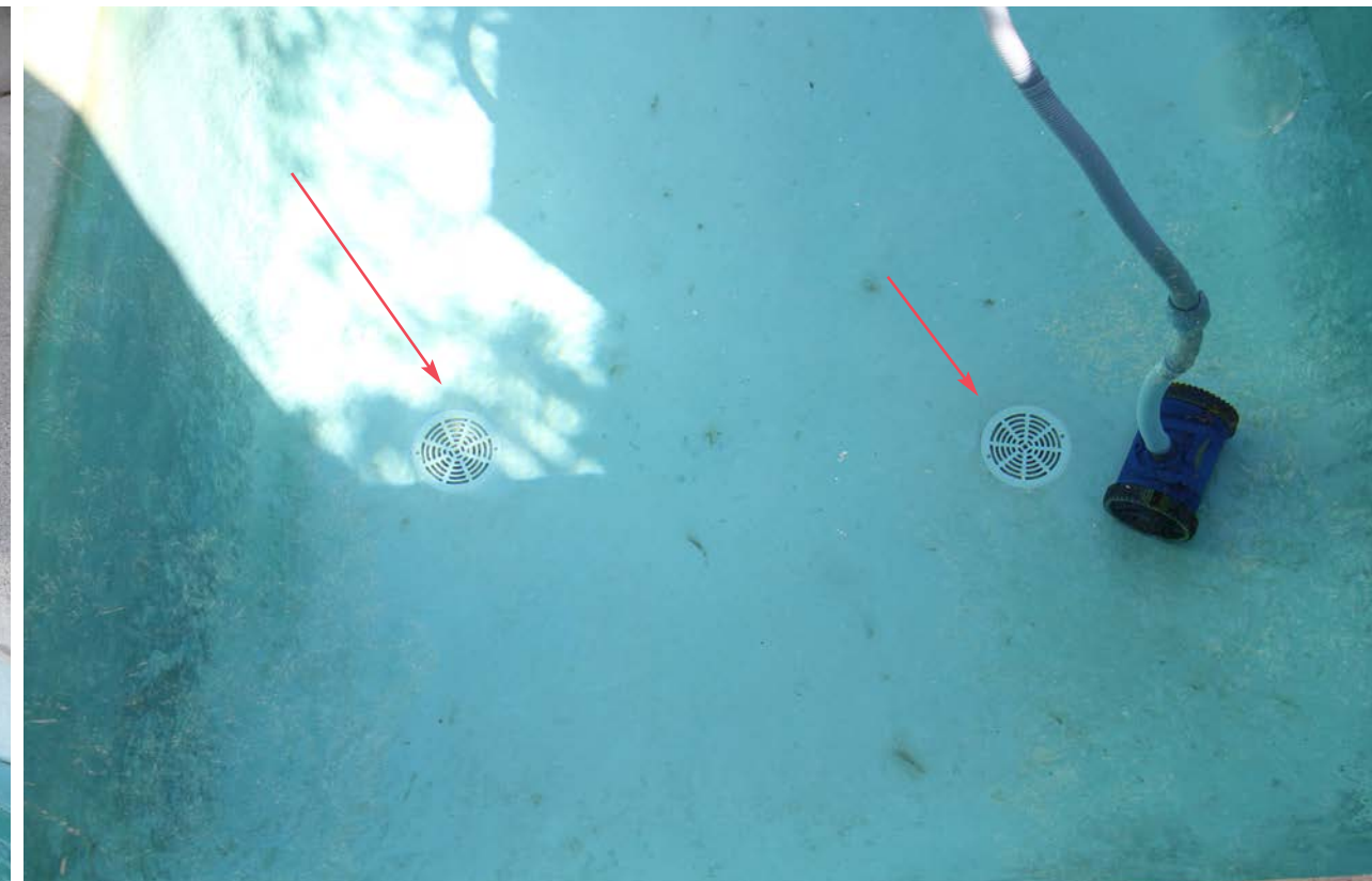
Two drains in deep end for safety, with pool sweep
