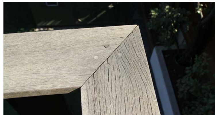
Mitered corner with sunken screws and tapered plugs
