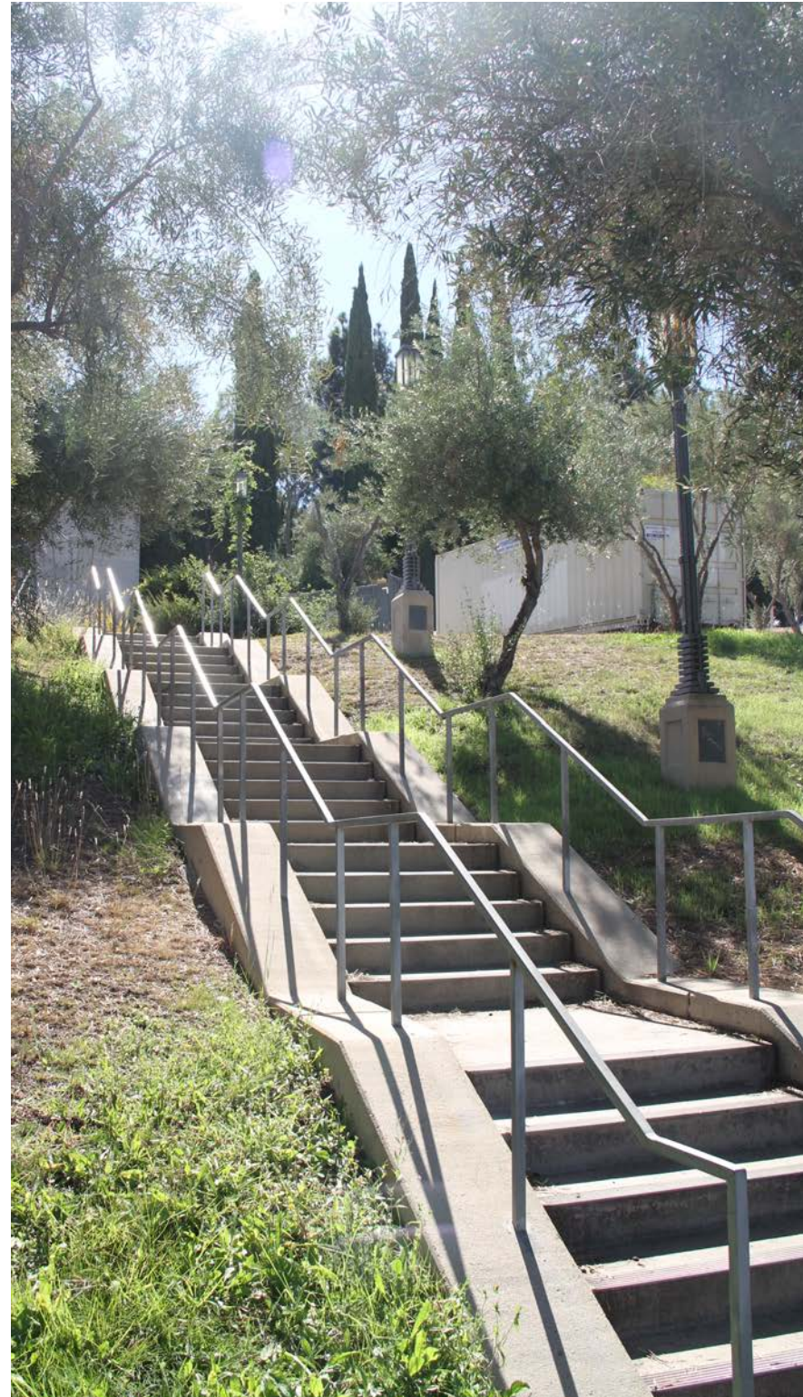
Steps and handrails (to code) at Barnsdall Park. Newly constructed (1995).
