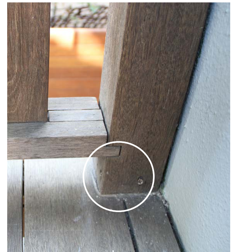
Screws at post base put in at 45 degree angle.
