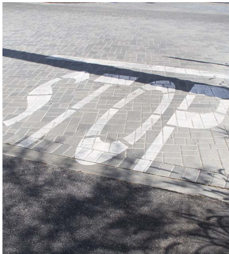
Interlocking paving stone with beveled edge, delineating intersection
