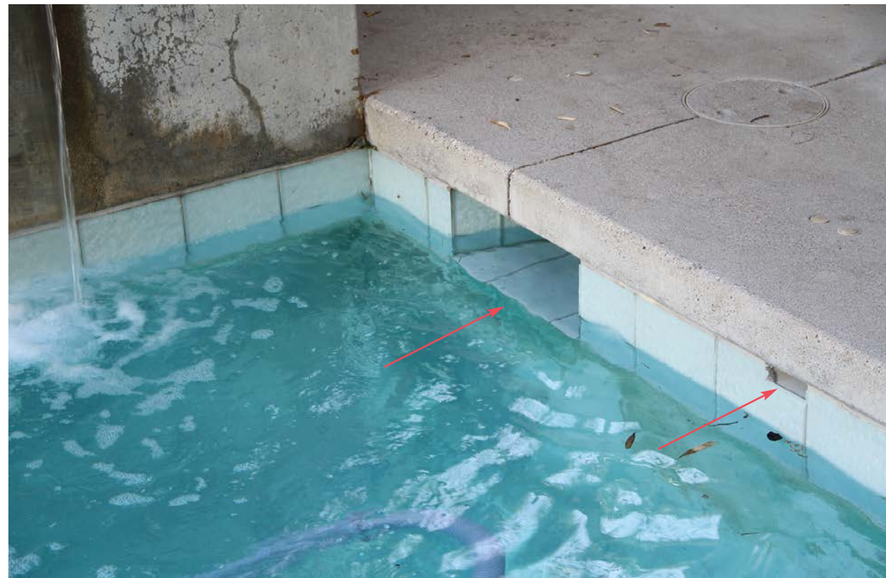
Skimmer in deep end. Small outlet, to the right, is a drain that goes straight to the street if it rains and the water in the pool overflows.
