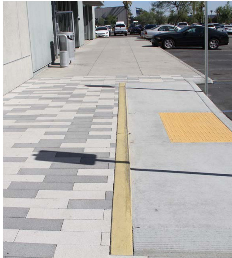
Flat granite paving stones, bordering ADA ramp, with expansion joints. 3' x 4' detectable warning surfacellanding in yellow at low point.
