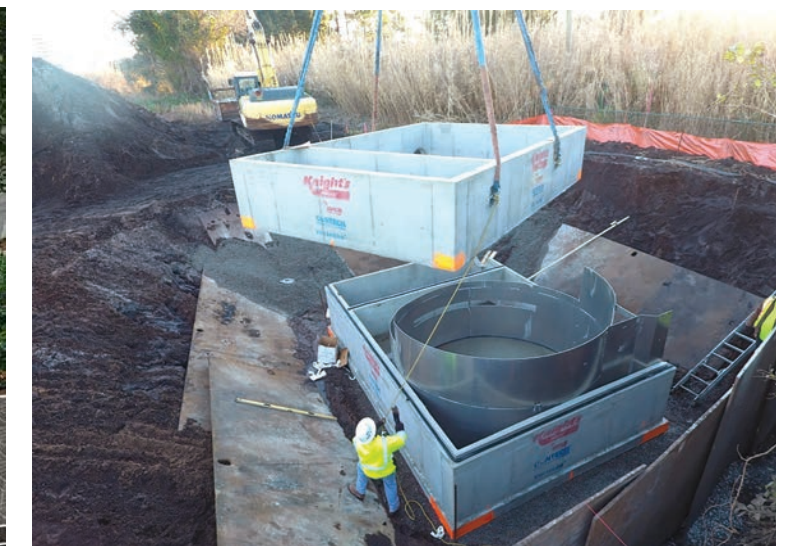
A vault-style hydrodynamic separator for treating stormwater runoff. This system combines swirl concentration and flow controls into a single unit for removing fine particles and other pollutants. It utilizes a four stage chamber design (swirl, floatables, flow control, and outlet chambers) with a special baffle and weir design to effectively remove sediment, litter, debris and hydrocarbons.
