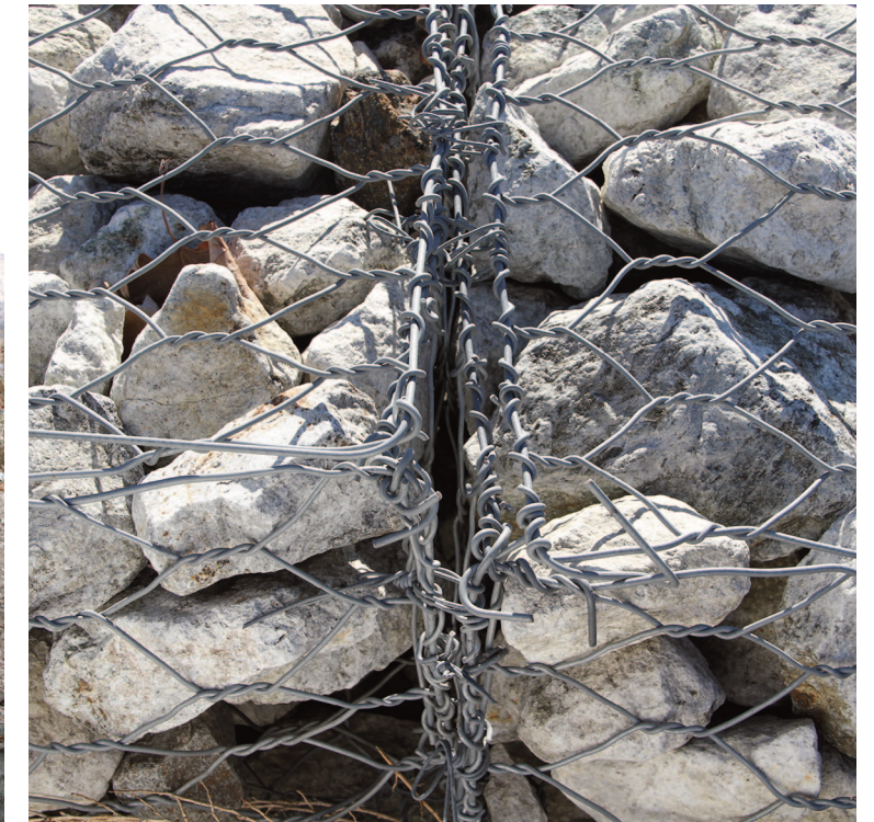
Detail of how the wire cubes are attached together.
