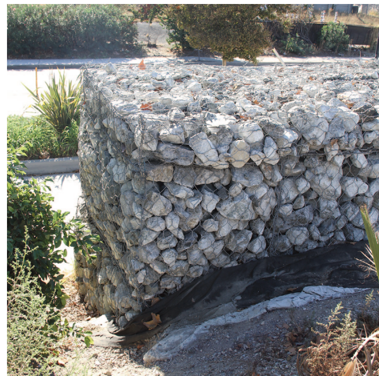
Detail of corner on the slope side. Most gabion retaining walls don't need concrete foundations. Depending on the wall height, a 2" to 4" layer of compacted 1" road base, crushed from either blue metal or basalt rock is all that is required for most gabion walls.
