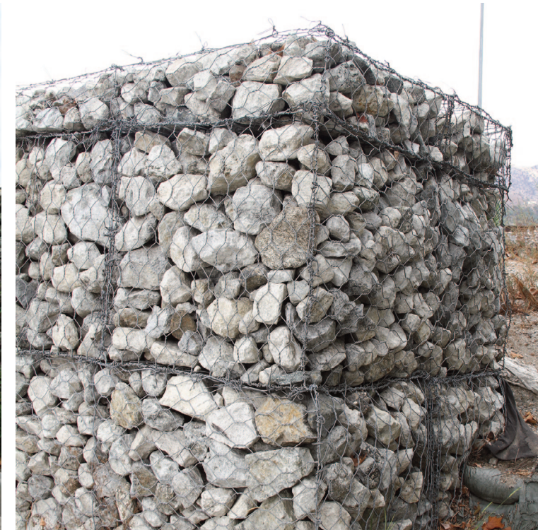
Corner detail showing the 36" wire cube cage with an additional 1' cap section at the top
