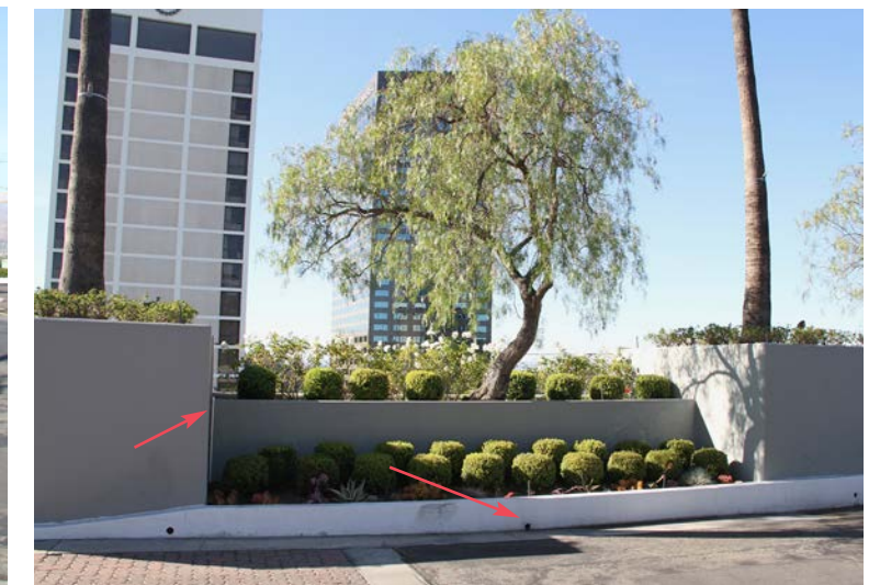
Lower tiered planter showing irrigation piping and weep holes for drainage.
