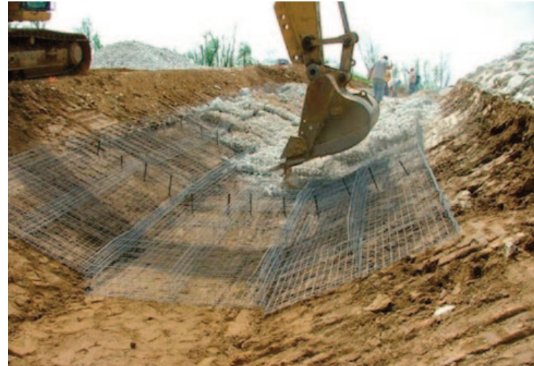
Filling the mattresses with stone.
