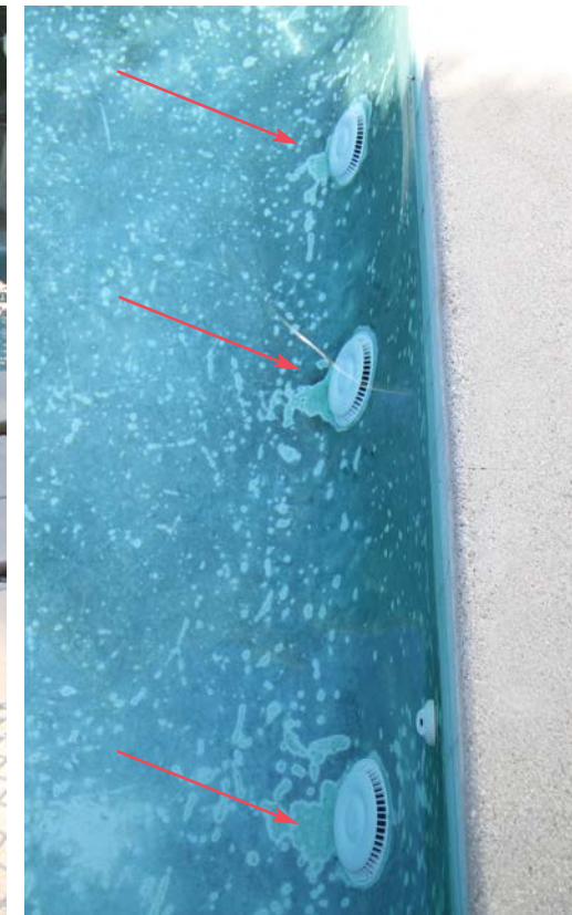
Outflow from filter equipment in shallow end
