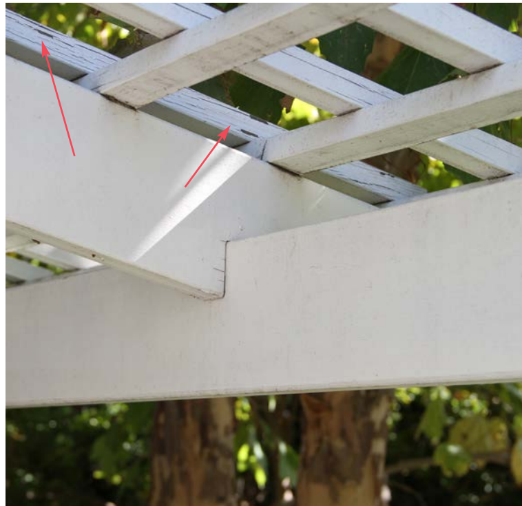
Wood splitting, stain chipping on top
