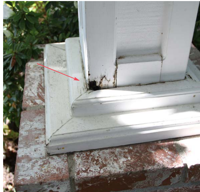
Base of column: Termite damage
