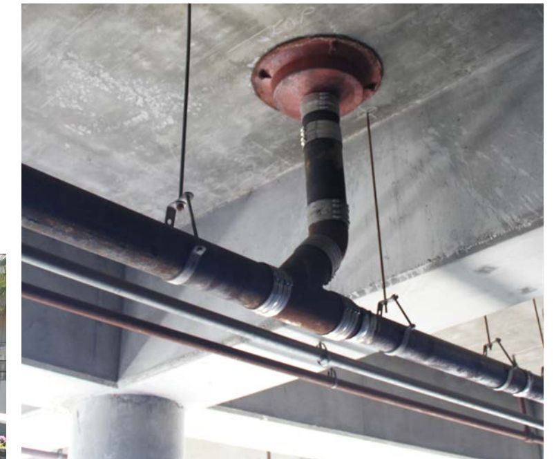
Drainage pipes under the planter boxes from level below in the parking garage
