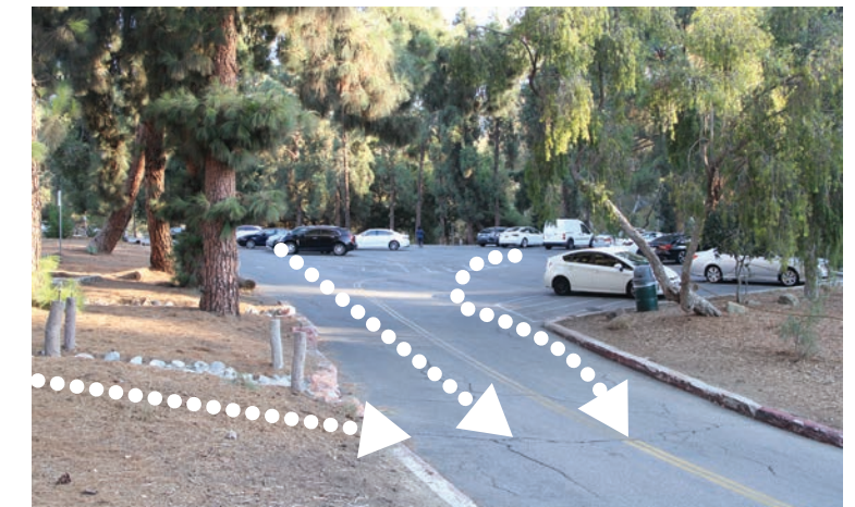
Highest elevation parking terrace. Should be outfitted with drains in permeable paving for feeding into lower elevation cistern.
