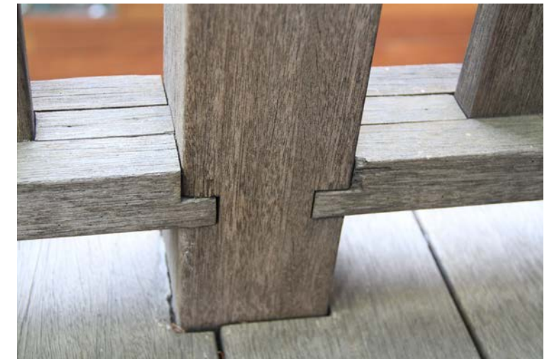
Slotted post where base rail connects
