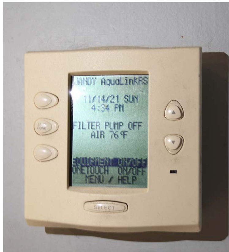
Pool controller inside the house
