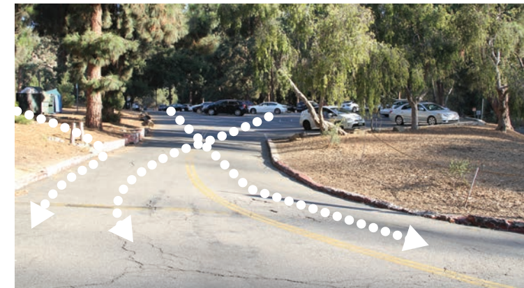
Slope of parking lot above cistern area showing elevation for water flow. Asphalt should be replaced with permeable paving. This water flows right into the dumpster area above.
