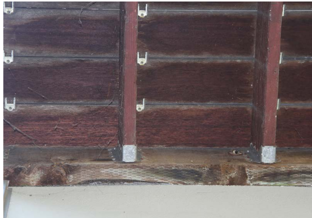
Joists connected to the ledger with metal joist hangers. The other metal objects are hidden deck fasteners, which are attached from above.
