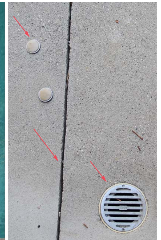
Covers for fence holes, expansion joint, walkway drain cover
