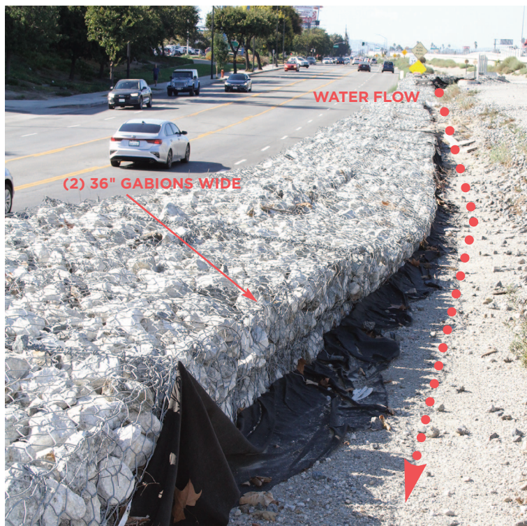
Top of the wall, (2) 36" cube cages wide, with the geotextile fabric against the slope. Top of gabions are sloped away from the street traffic. A channel has been created for drainage away from the street, and down towards the plantings and trees of the Animal Shelter property.
