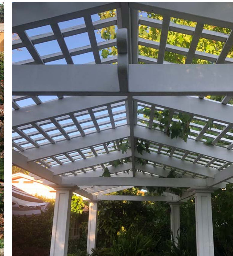
Inside roof detail
