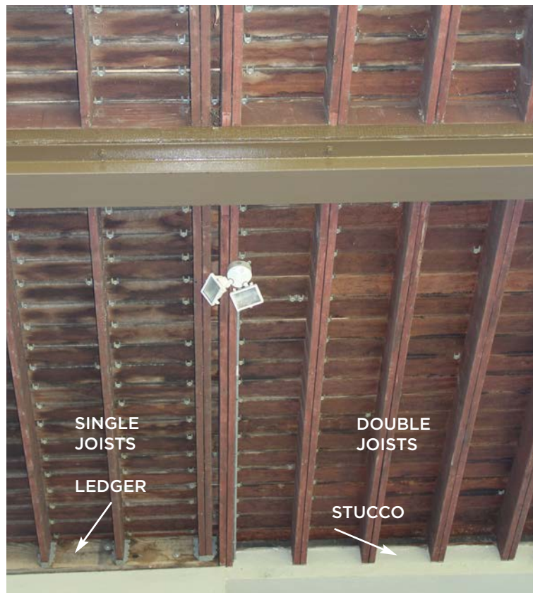
Single joists (attached to ledger) and double joists attached to balcony supports that are original to the house.
