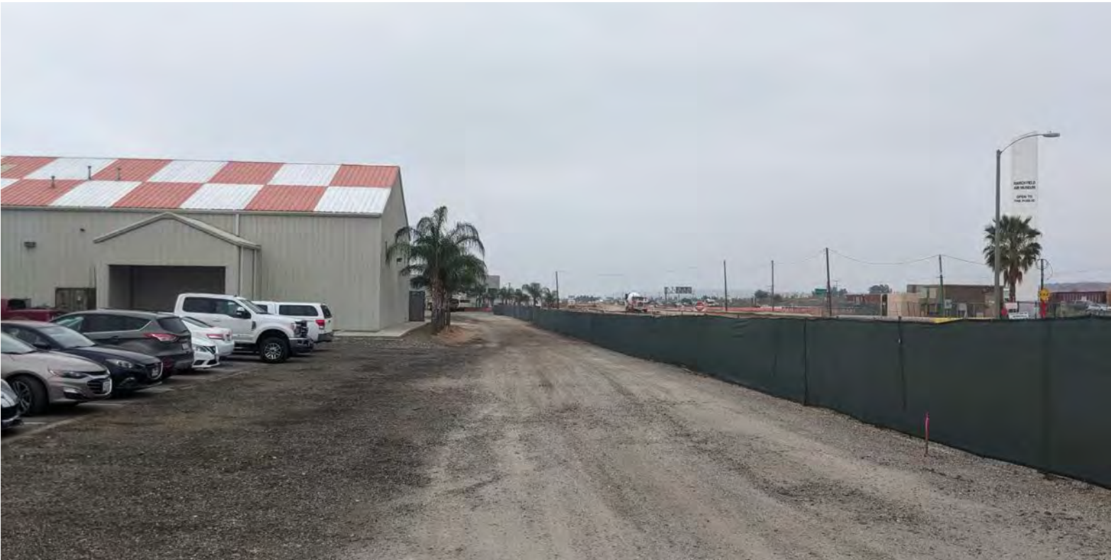
Staff parking, Van Buren Boulevard construction at right
