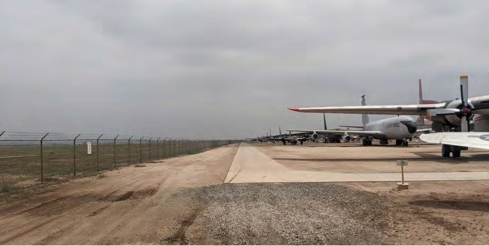
Perimeter near airfield
