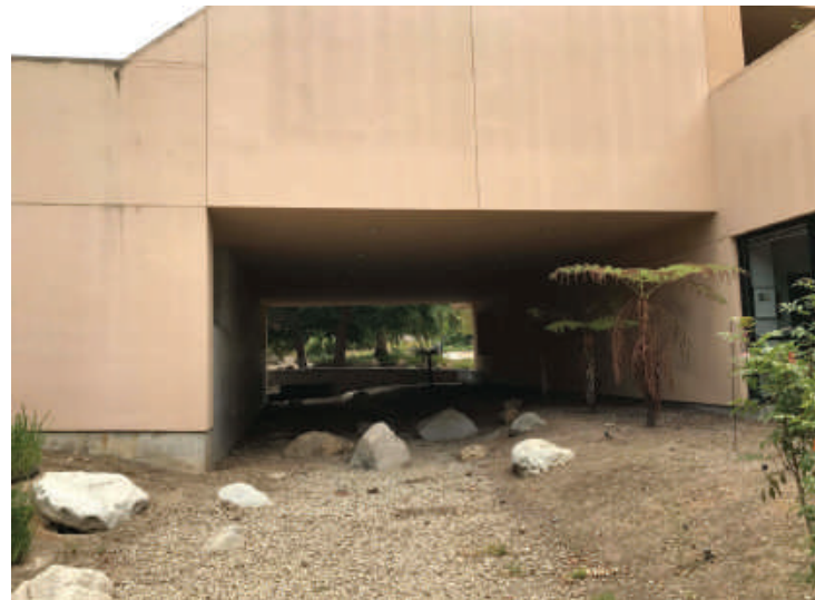
Drainage swale passes under building
