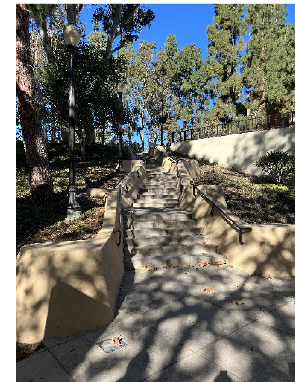
VIEW NW FROM BOTTOM OF STAIRS
