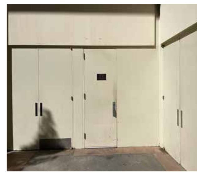
Many outward swinging doors on all walls, disrupting available usable space
