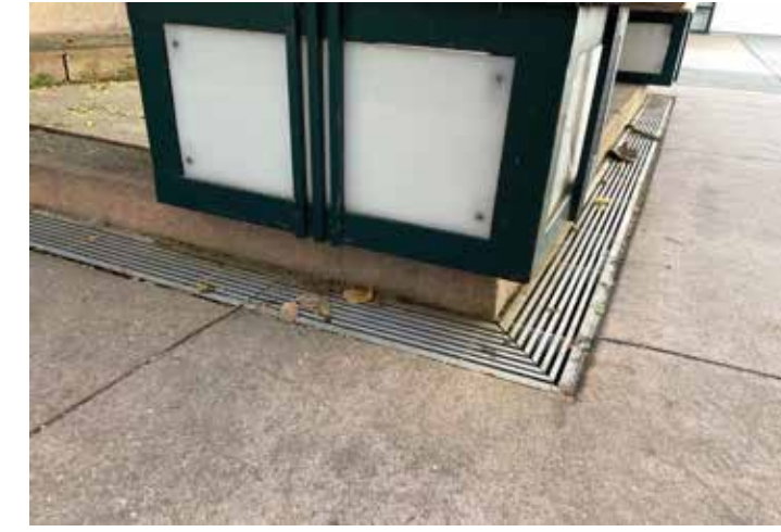
Center of courtyard drain inlet
