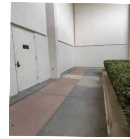
Highest point, NW corner, sloping into first planter and drain inlet and towards center of courtyard, Outward swinging door and outlet
