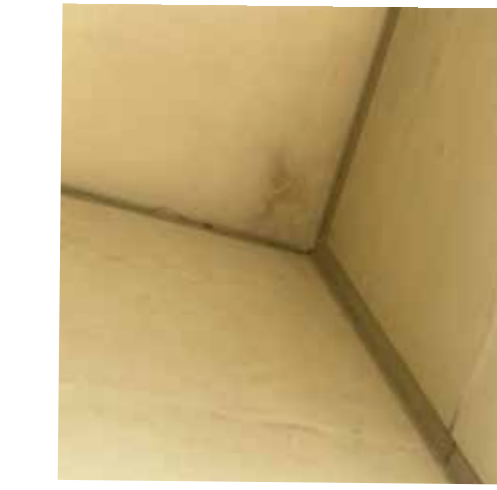
Crack along N of ceiling with water damage on NE corner
