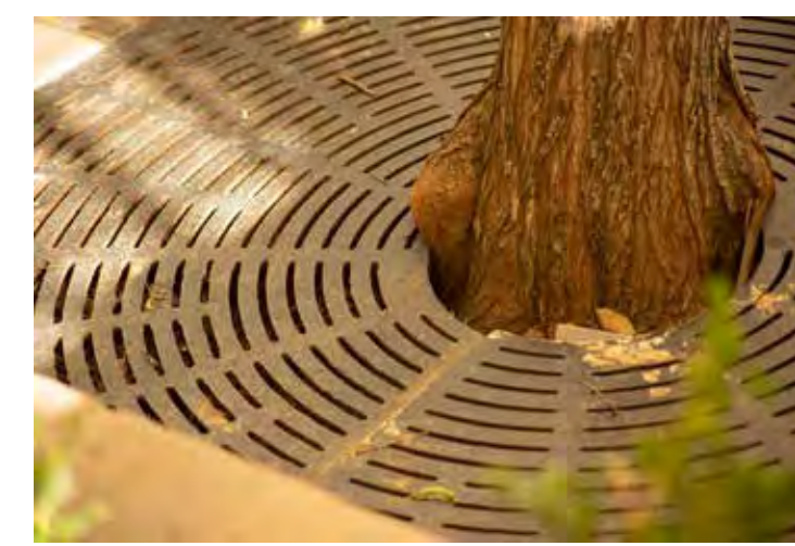
Drainage grate constricting a tree on west side of courtyard
