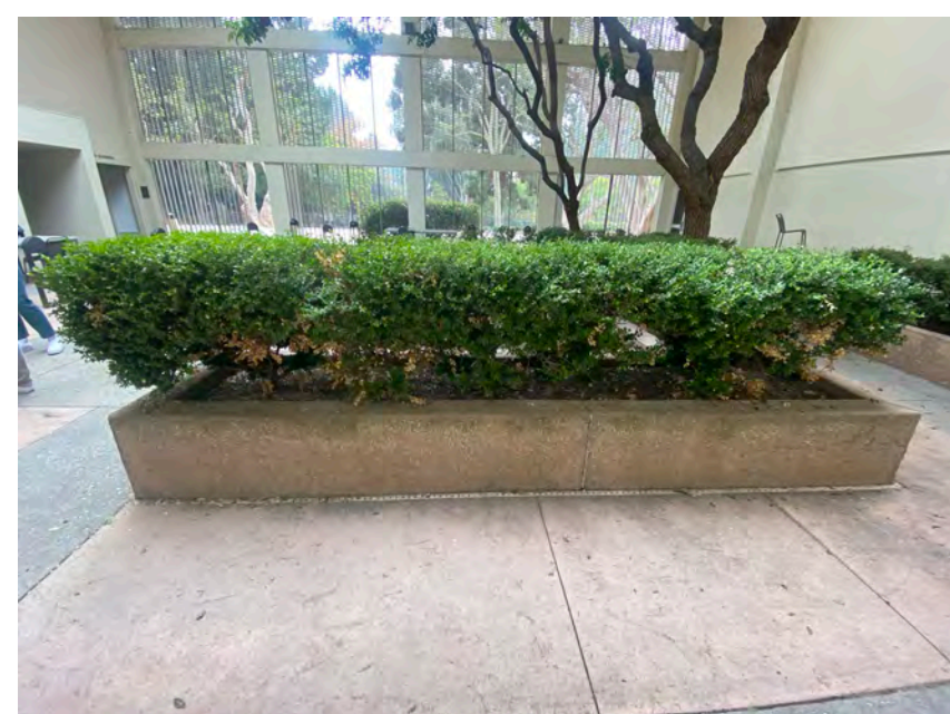
HARDSCAPE CAN'T ABSORB RAIN THAT FALLS THROUGH SKYLIGHT
