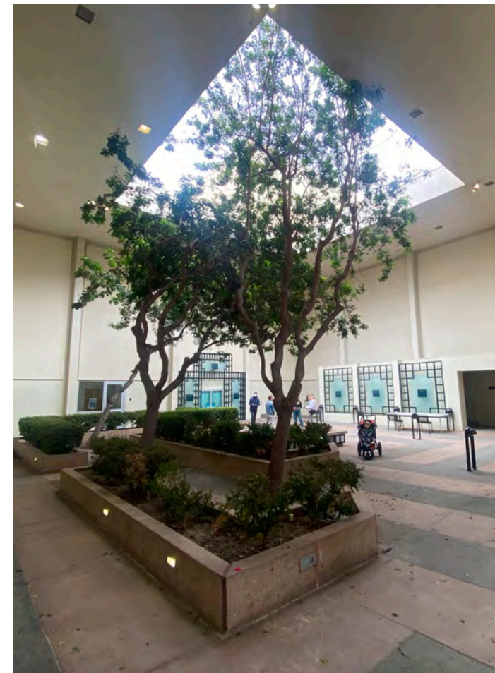
SKYLIGHT SPLASH ZONE TOO MUCH HARDSCAPE
