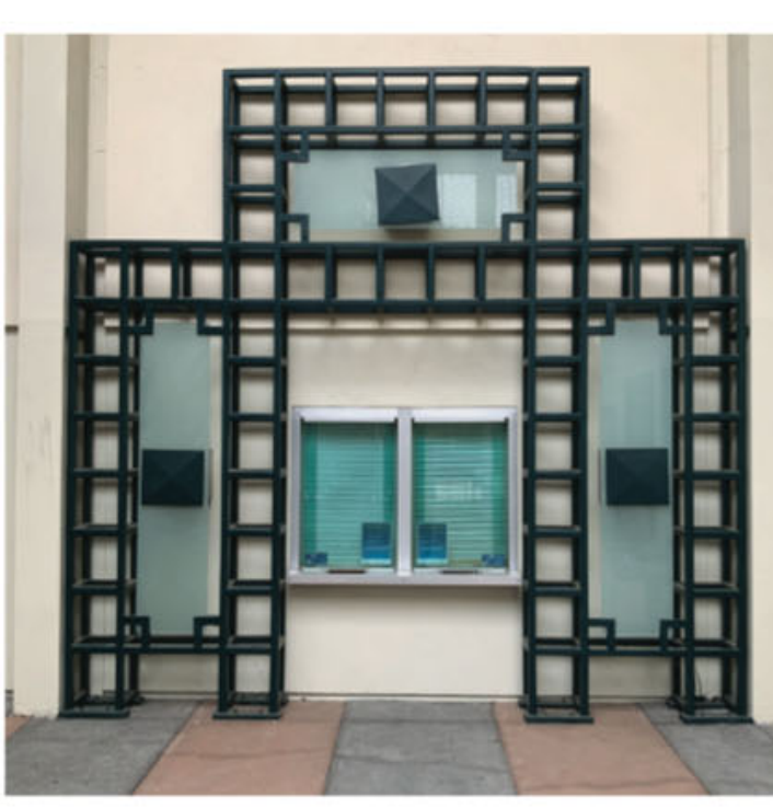
WALL TREATMENT AT TICKET WINDOW
