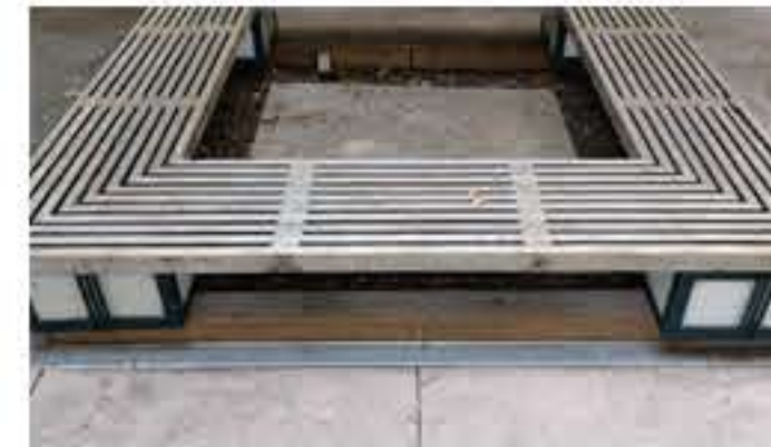
G. DRAINAGE AROUND WOODEN BENCH. LIGHTS ON EACH CORNER. BENCH LATER ADDITION.
