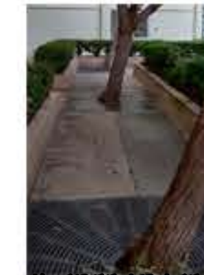
H. TREE GRATE & DRAIN ALONG PLANTER.
