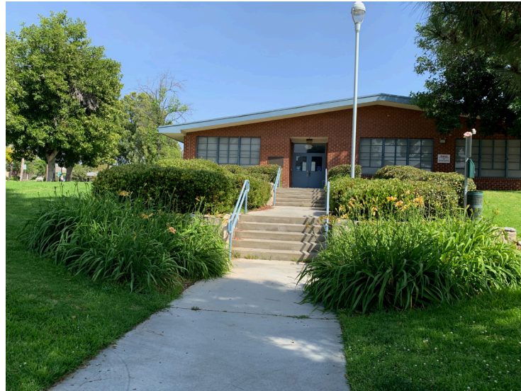
4 Looking NE at topo & existing community center - proposed site
