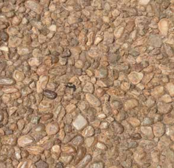
Integral colored exposed aggregate concrete paving
