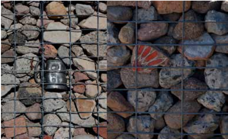
Example of gabion filled with recycled materials. Photo Credit: Landscapeperformance.org
