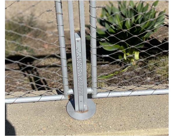
PATH LIGHTING ON RAMP FENCING
