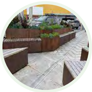
Sand Finish Concrete With 6' Scorelines
