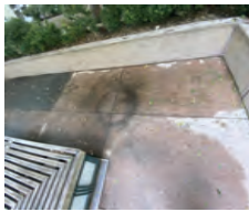
Moisture collects in puddles: needs adequate and well-placed drainage
