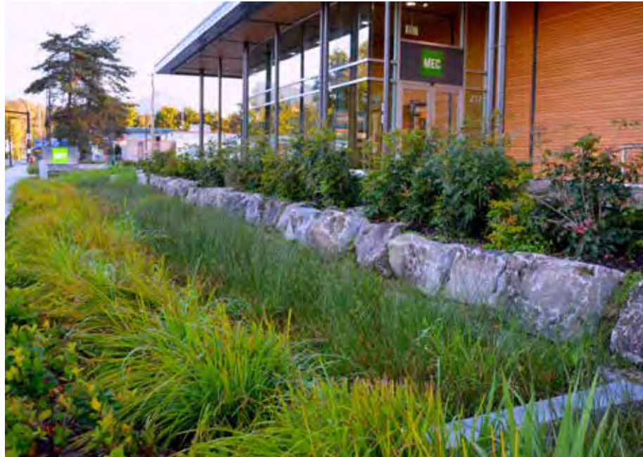
Depths of rain gardens can vary from 6" to a few feet depending on location and amount of stormwater capture needed for the site.
