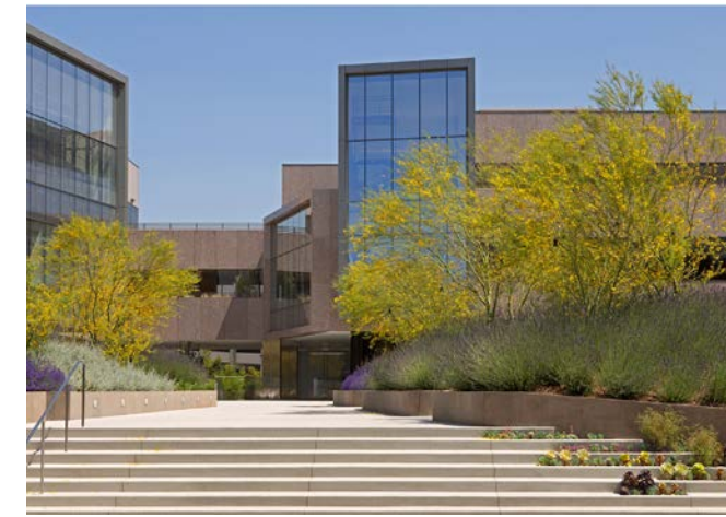
Visually clear building entrance
