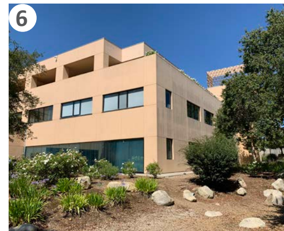
6 View of City Hall office windows. Photo was taken facing West while standing in dry creek bed.
