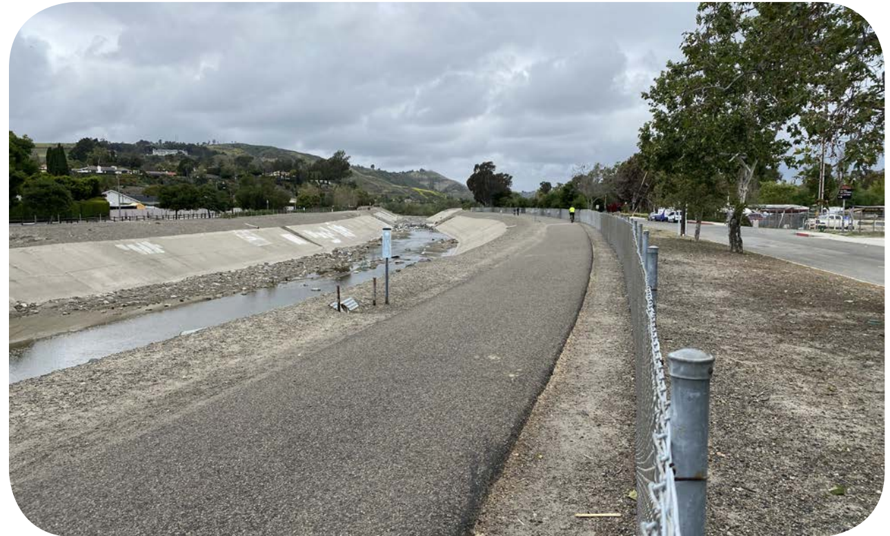
1 Trabuco Creek concrete channel and bike path facing north. No vegetation or suitable habitat.
