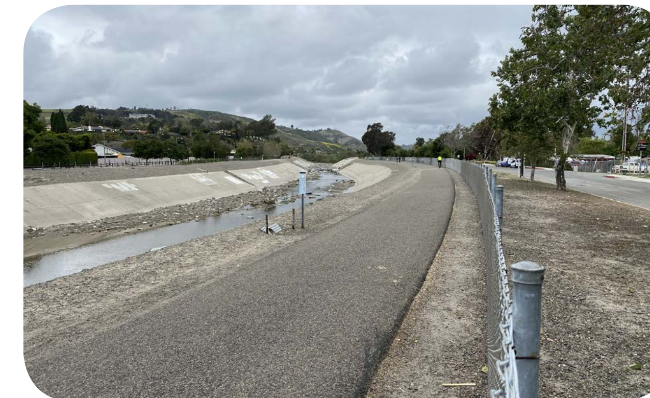
① Trabuco Creek concrete channel and bike path facing north. No vegetation or suitable habitat.
