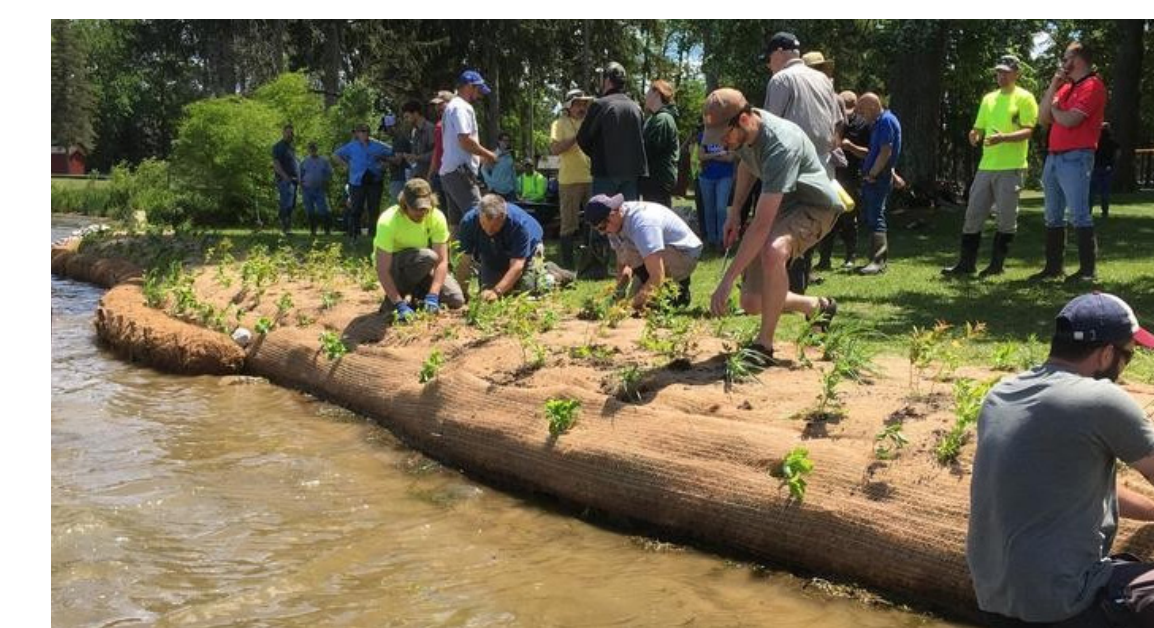
WETLAND RESTORATION | USACE Bioengineering Techniques
